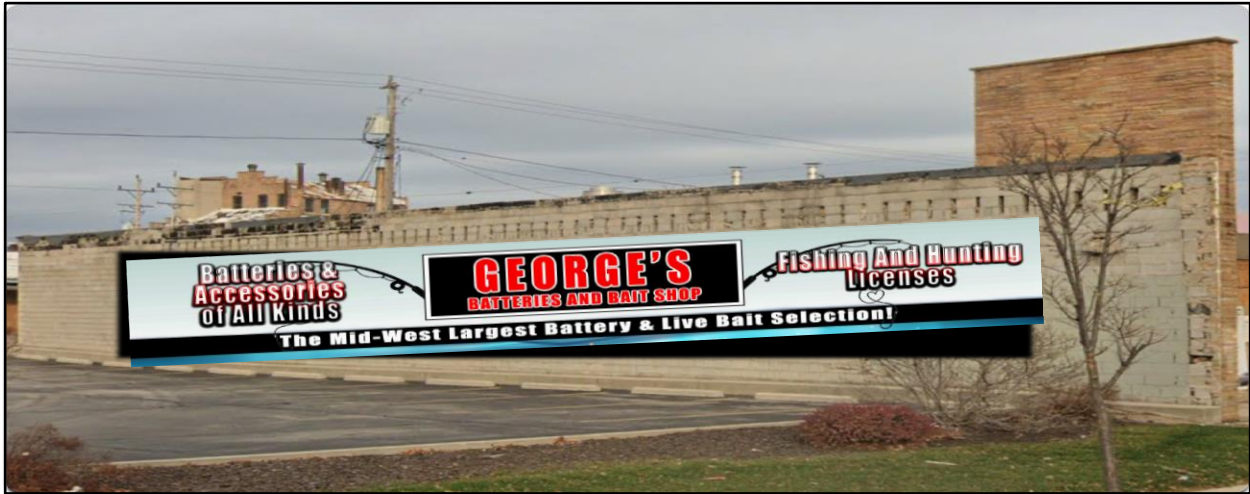
LETTERING ON SOUTH SIDE ENTRANCE AND PAINTED SIGN FOR BUSINESS ON WEST SIDE OF PROPERTY.
