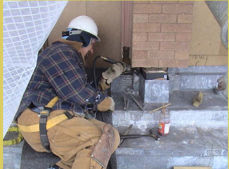
Continued soldering of lead-coated copper through wall flashing.
