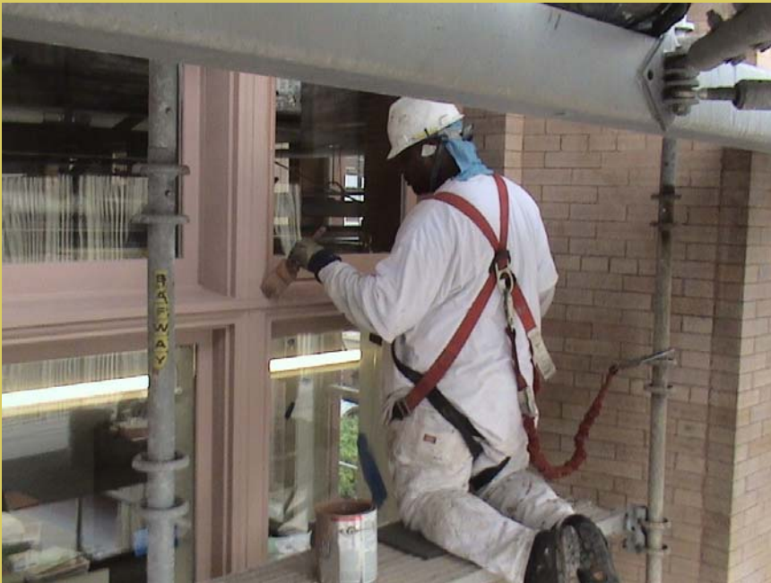
Painter applying finish coat of paint on the exterior window frames.
