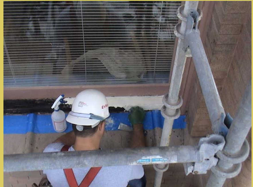
Repairing of wood window sills.
