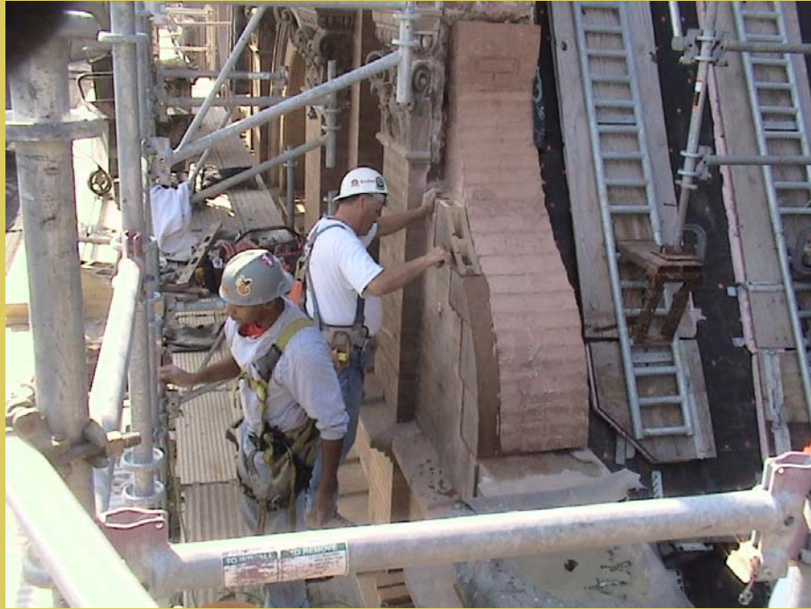
Installing the new stepped terra cotta pieces
