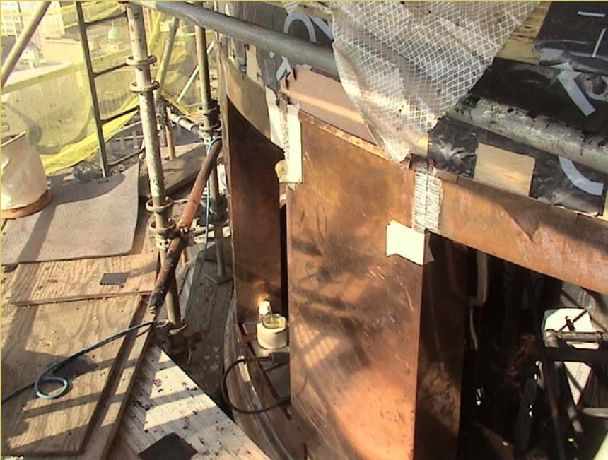
Red copper cladding around drum of south tower.
