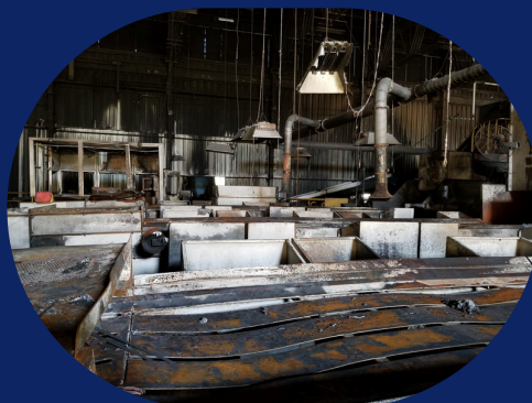
Sorting floor post-fire
