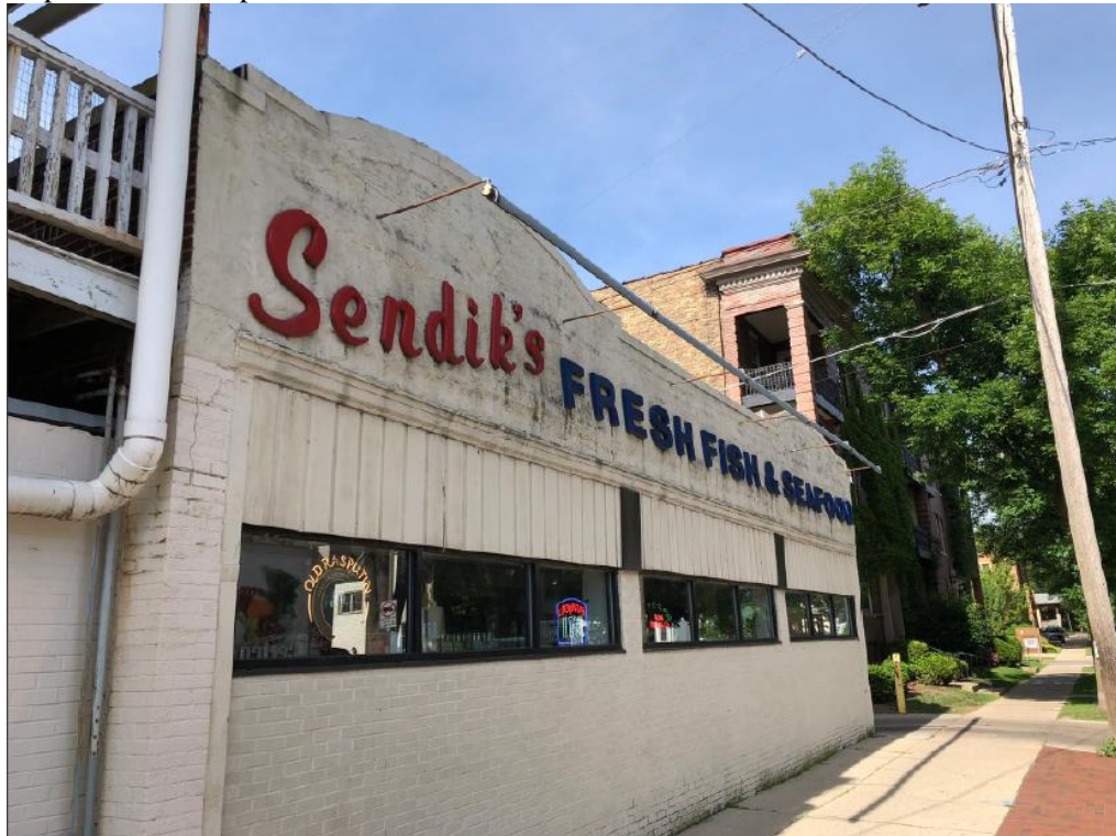
Affected elevation before start of work.
