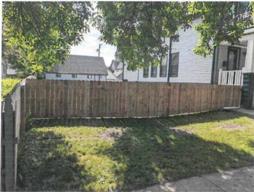
Street view of fence on north side of house
