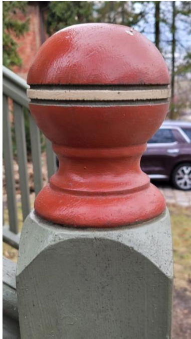
Existing Post Finial (Front Porch)
