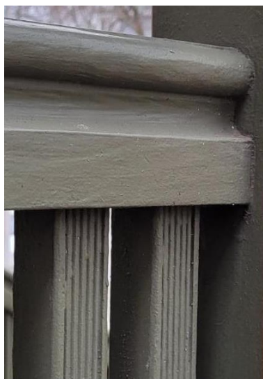
Existing Handrail (Front Porch)
