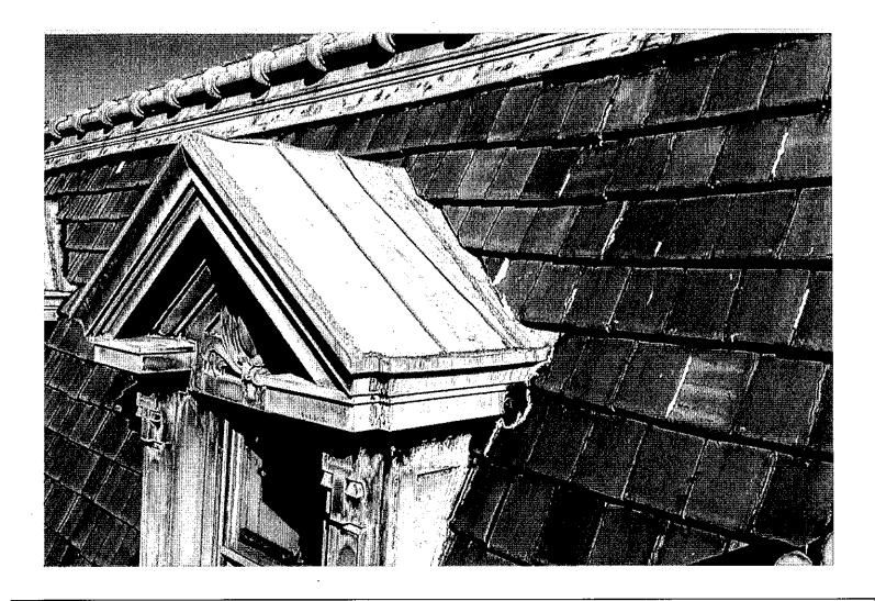
Original roof tiles are spalling and cracking. They will be replaced with new tiles that match as closely as possible. All fine copper detail to be retained or replicated if necessary.
