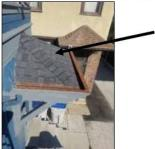
26. We will furnish and install one layer of ice and water shield to completely cover the entire roof area prior to the shingle installation.
