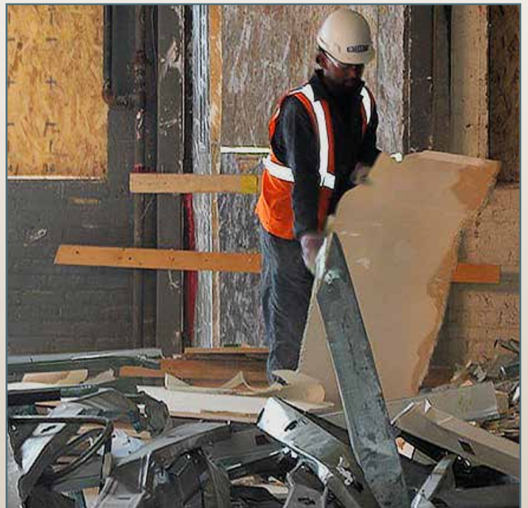
Worker removing debris.
