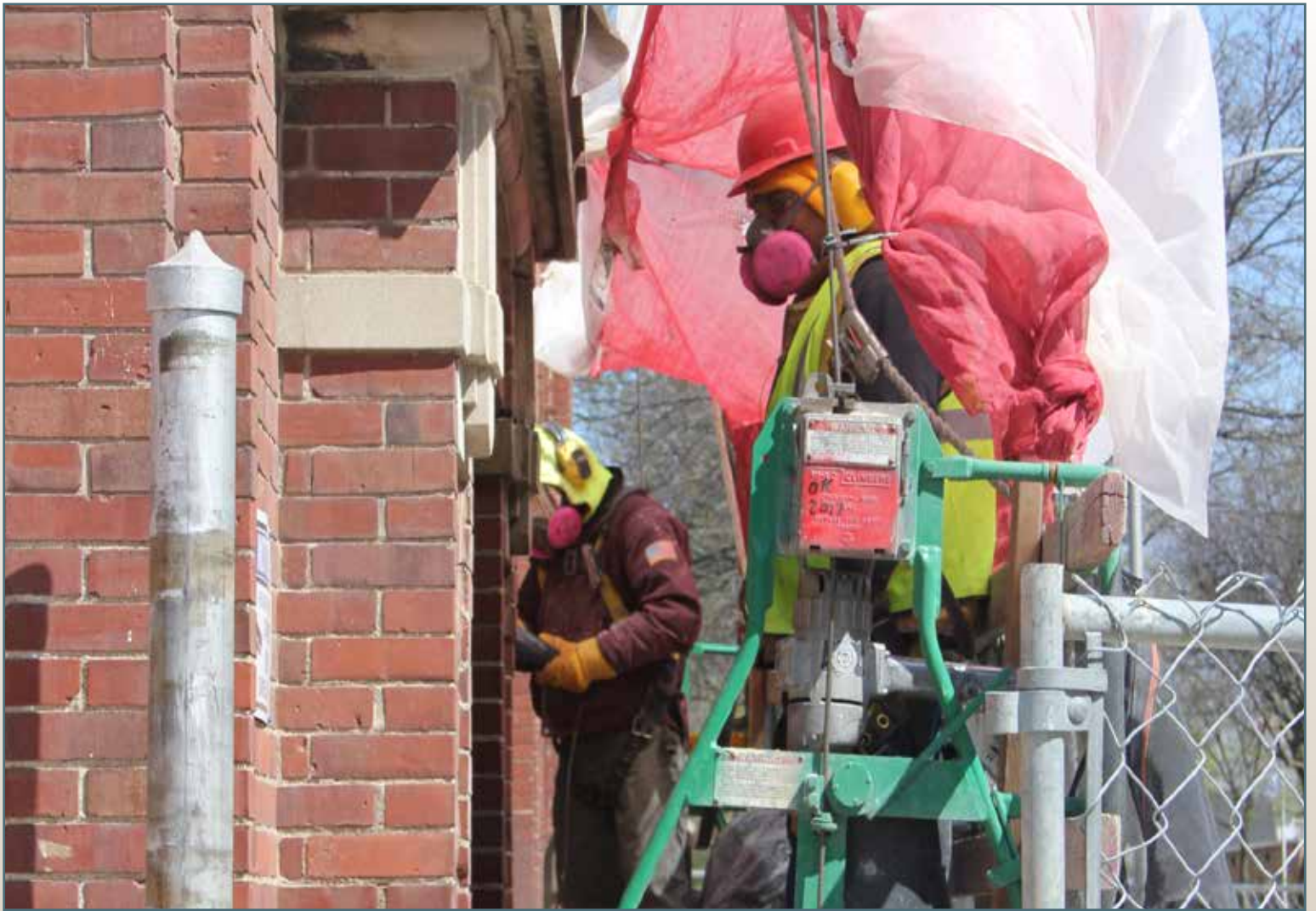
Workers removing asbestos.
