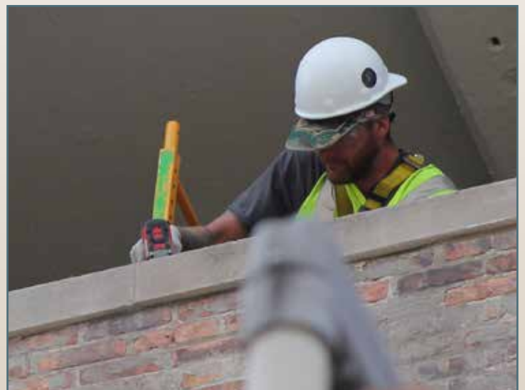
Worker preparing window installation.
