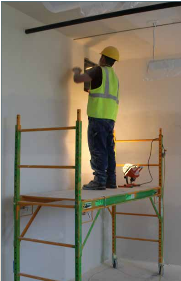
Worker finishing drywall.
