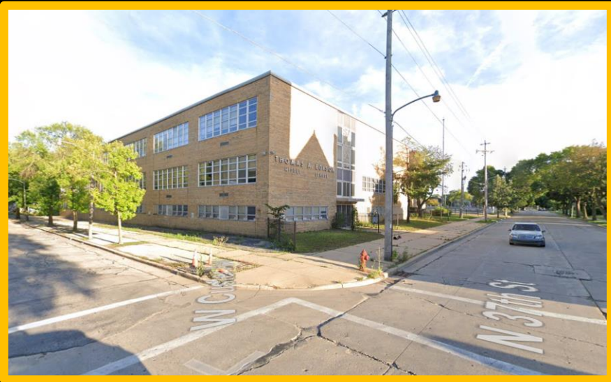
View from W Custer Ave and N 37th St looking south-east
