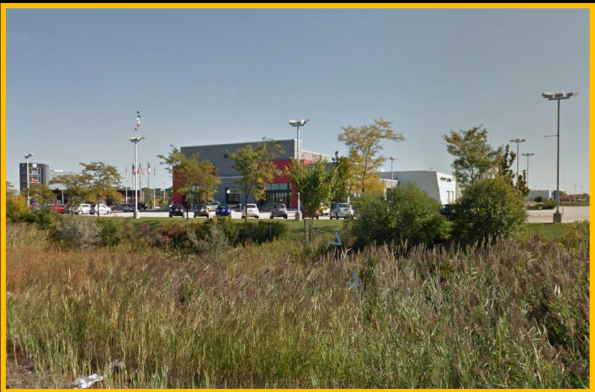
View from Interstate 41 off-ramp, looking northeast
