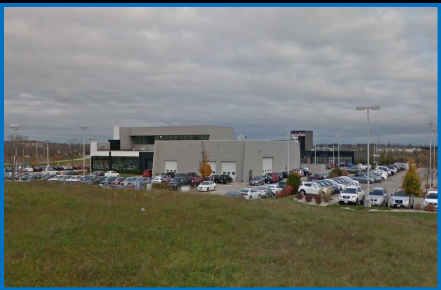
View from West Metro Auto Mall, looking northwest
