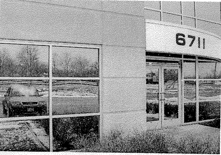
NORTH FACADE DETAIL OF PHASE I
