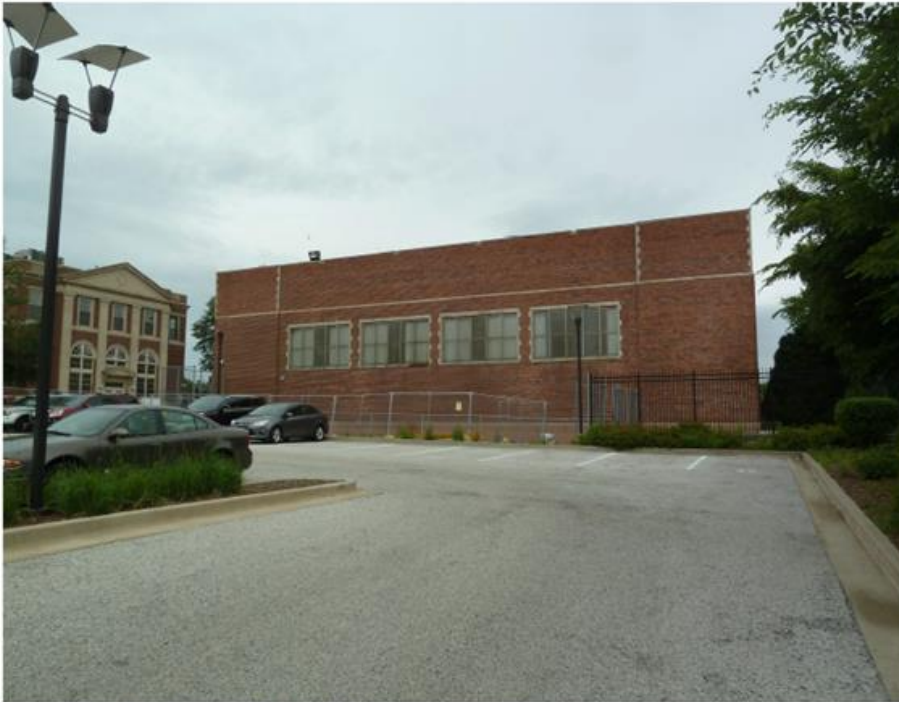
Photo 21 - North Overall at Pool Addition
