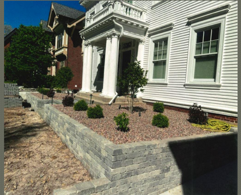
After manufactured stone; steps removed
