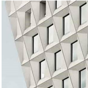
PRE-CAST PANEL/METAL PANEL
