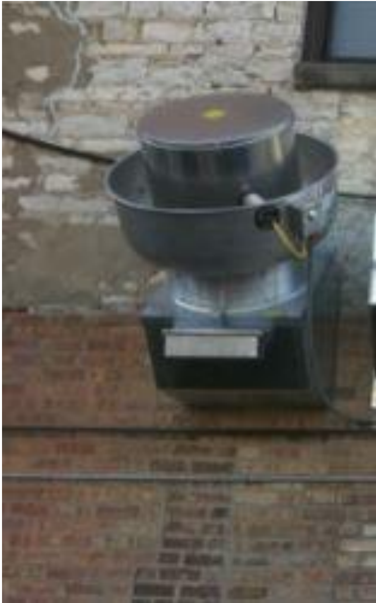
Image of the type of hood to be installed by Walters Sheet Metal
