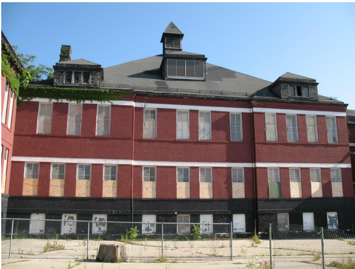
South elevation of 1888 addition
