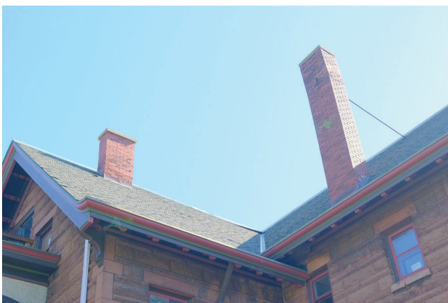
IMAGE 9: North and south chimneys with tie rod anchoring the south chimney.
