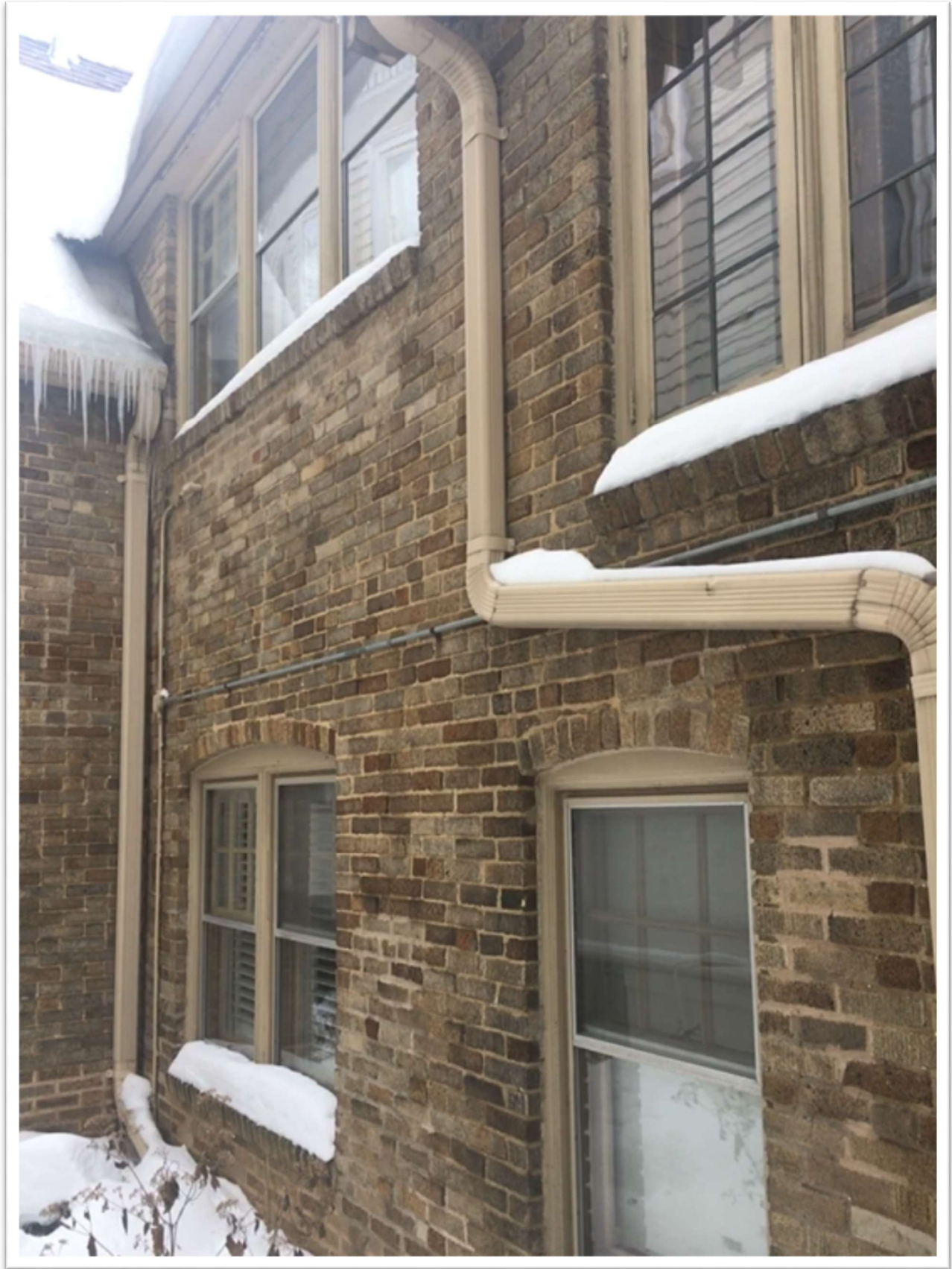
Figure 8. Some of storm/screen combinations to be replaced on west elevation.
