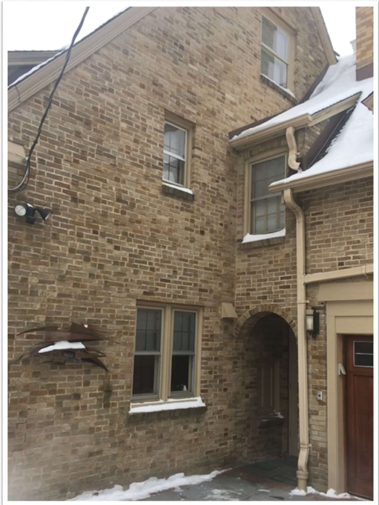
Figure 9. Some of storm/screen combinations to be replaced on north and east elevations.
