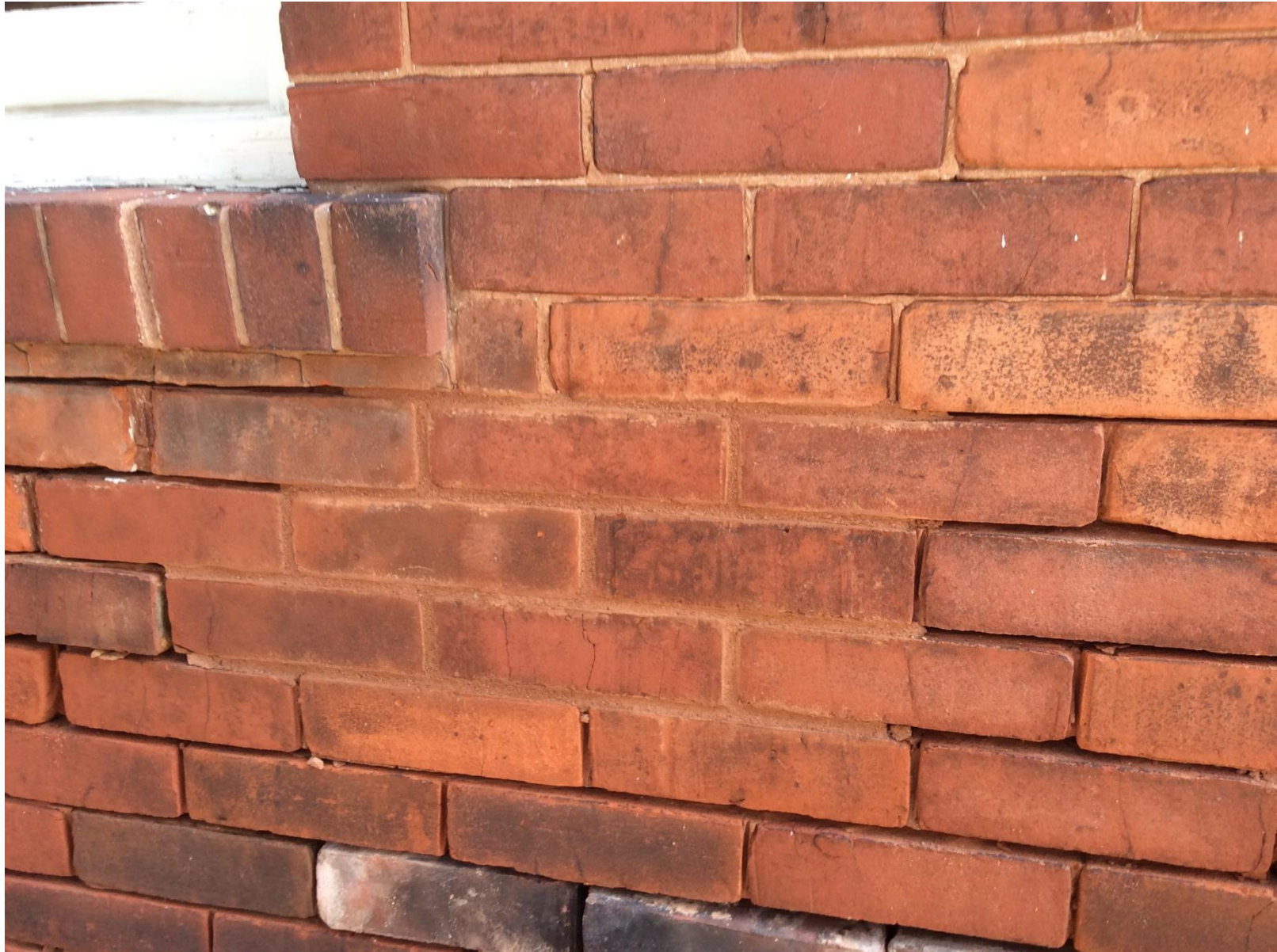
Mortar color sample is approved. Flush joints shall be used.
