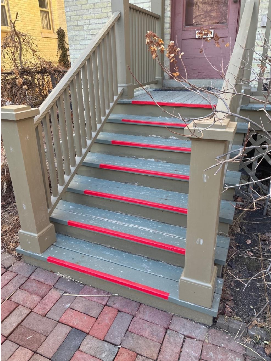
1031 E Ogden Ave Rear Porch
