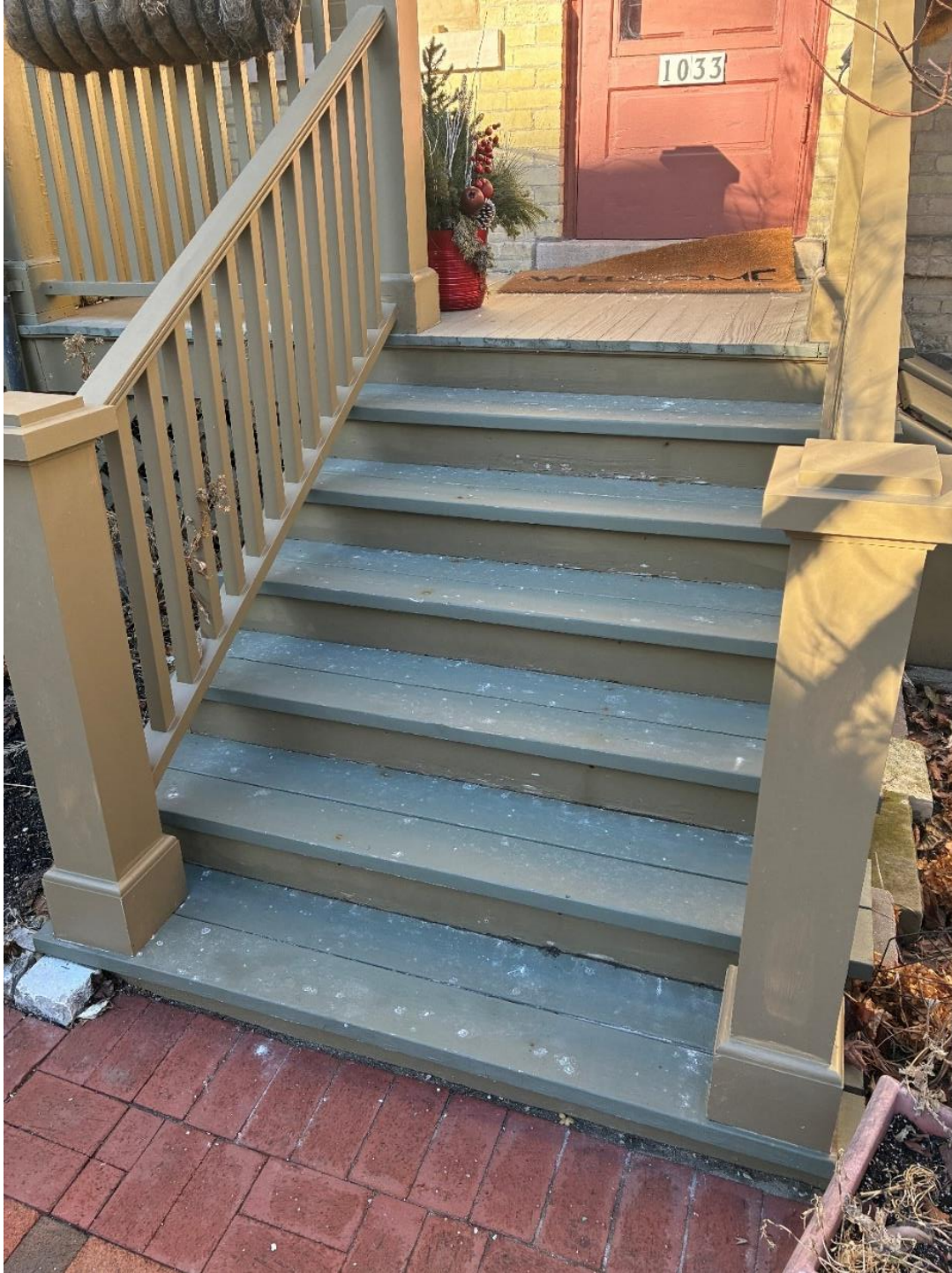
1033 E Ogden Ave Rear Porch
