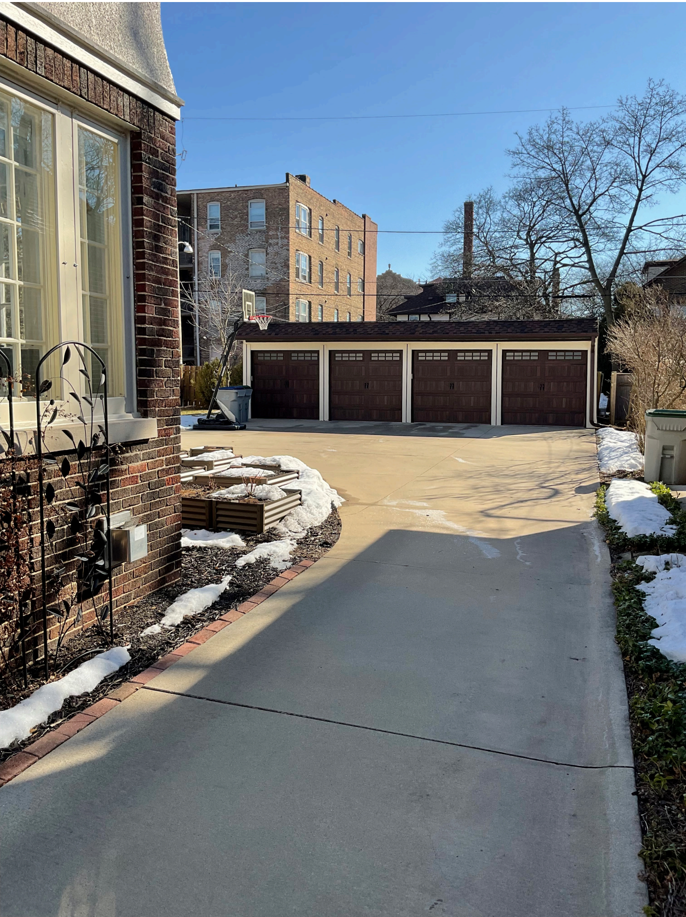
South side - rear yard & driveway side
