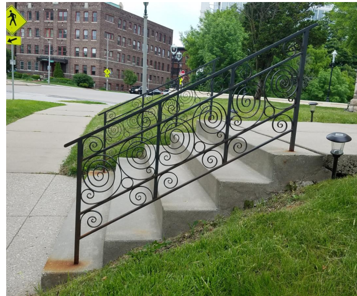
8 EXISTING STAIR RAILING
