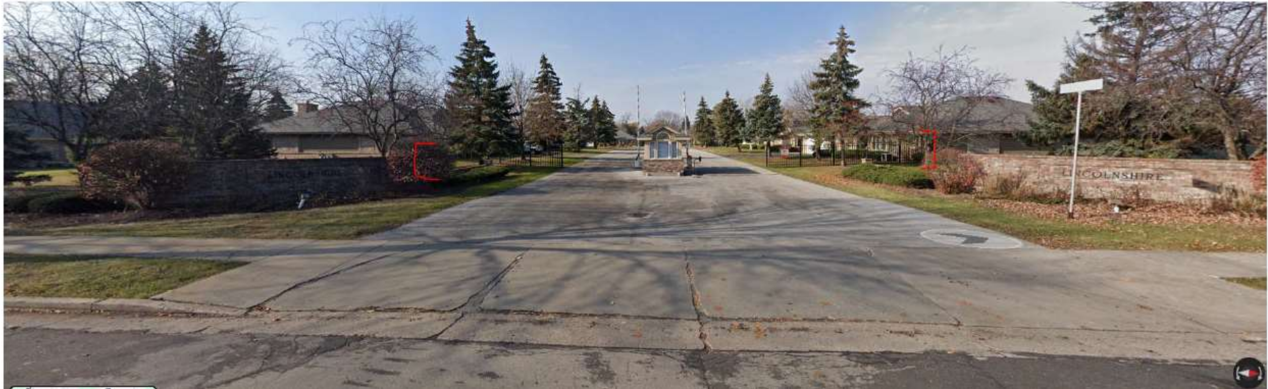
Images from Google Street View (Nov. 2021) – existing gate, gate house, and single arm barrier gates
