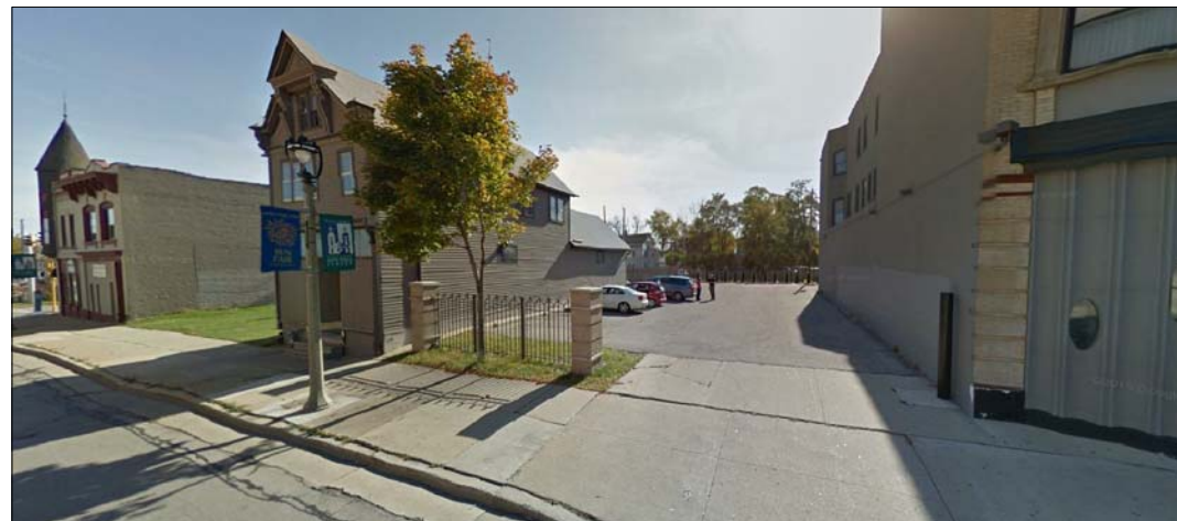
Existing Site Condition
