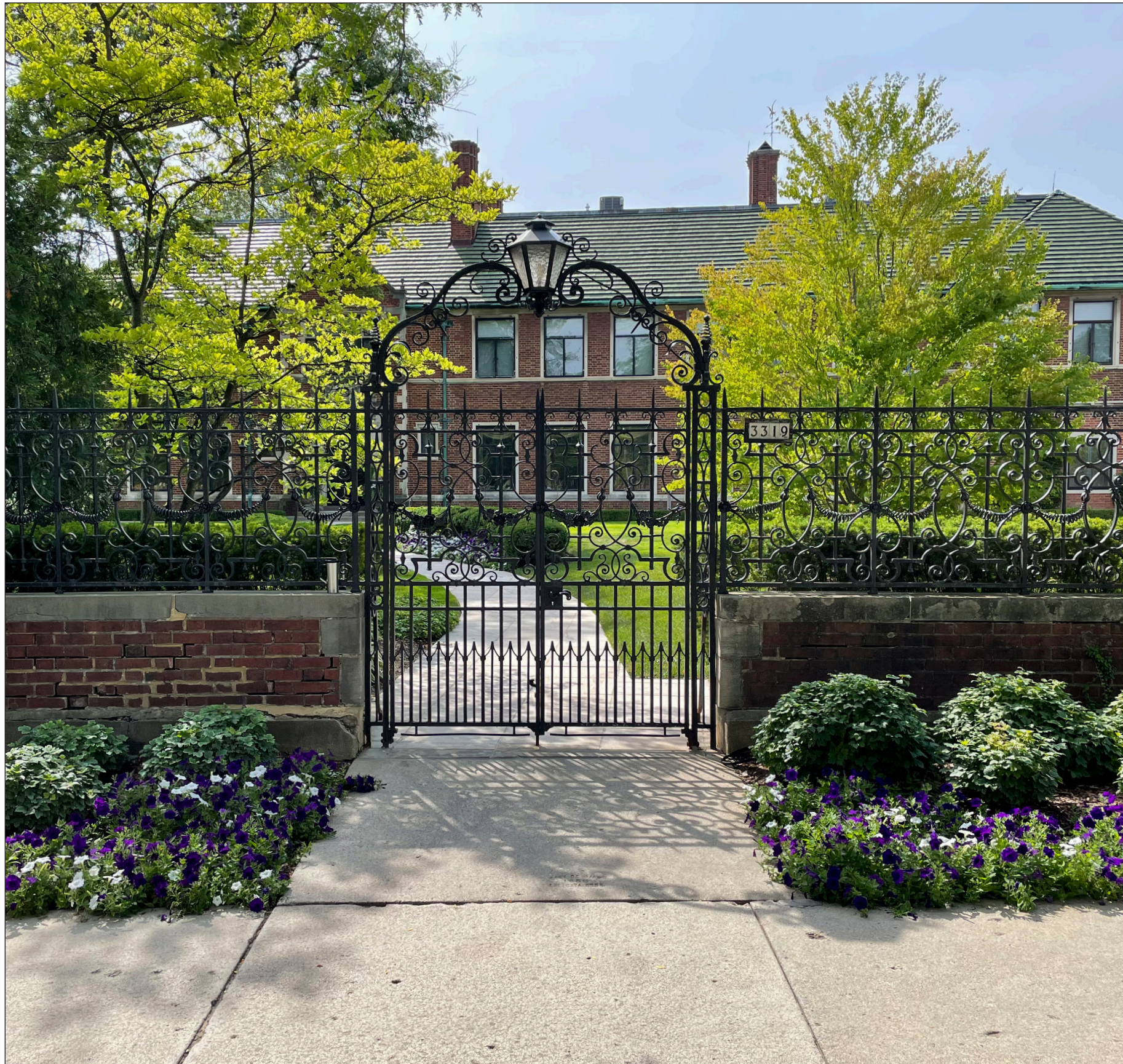
Lake Drive Entry - East Facade
