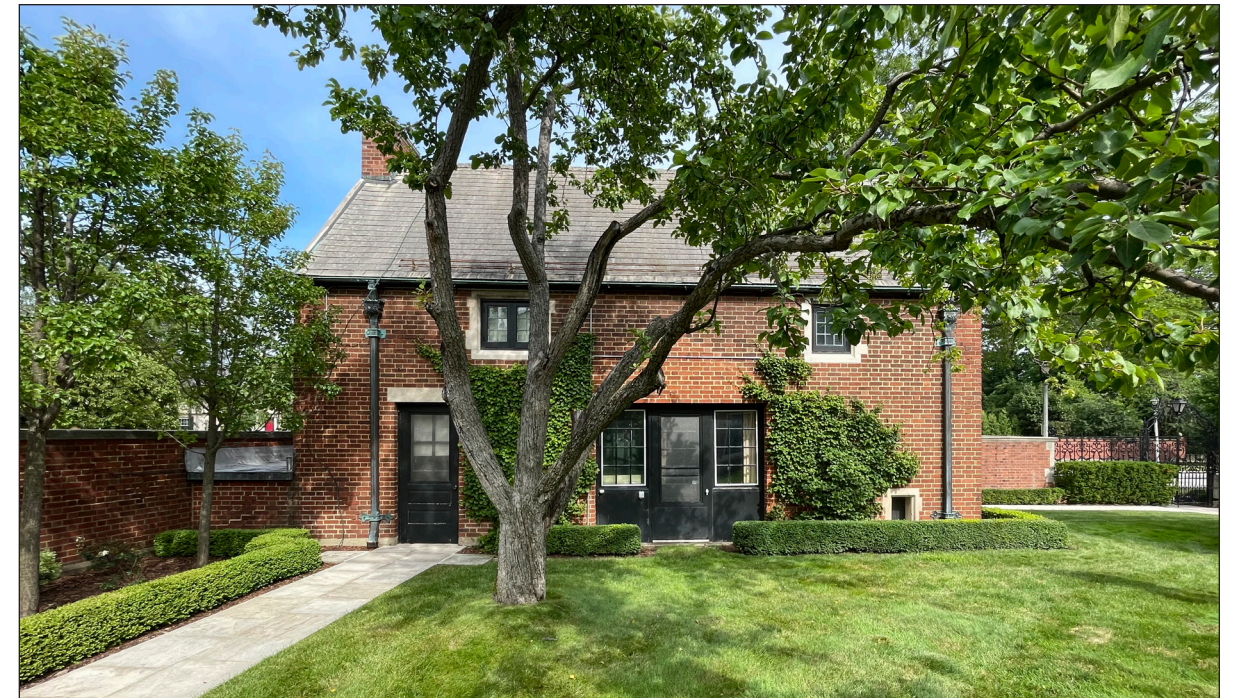
Caretaker's Cottage - West Elevation
