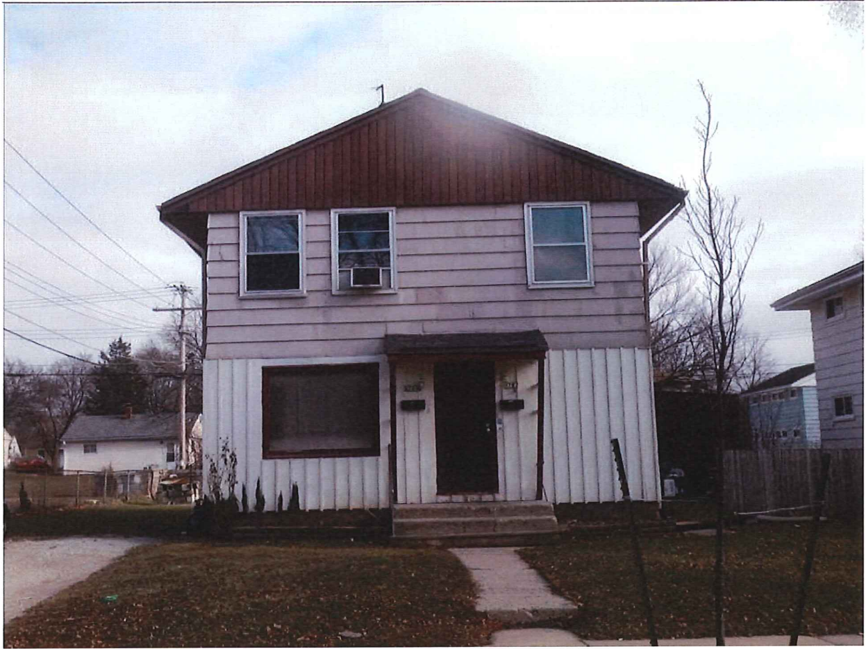
5700-02 North 61 st Street
