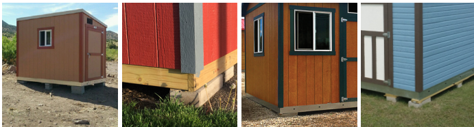
Sheds that have been leveled using concrete blocks and wood shims on a variety of surfaces and in a range of leveling severity.
