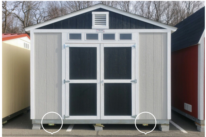
Figure 3 - Display building with wood skids beneath the floor joists
