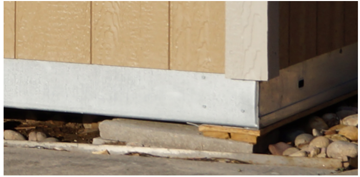
Figure 2 - Close-up of leveling with blocks & shims
