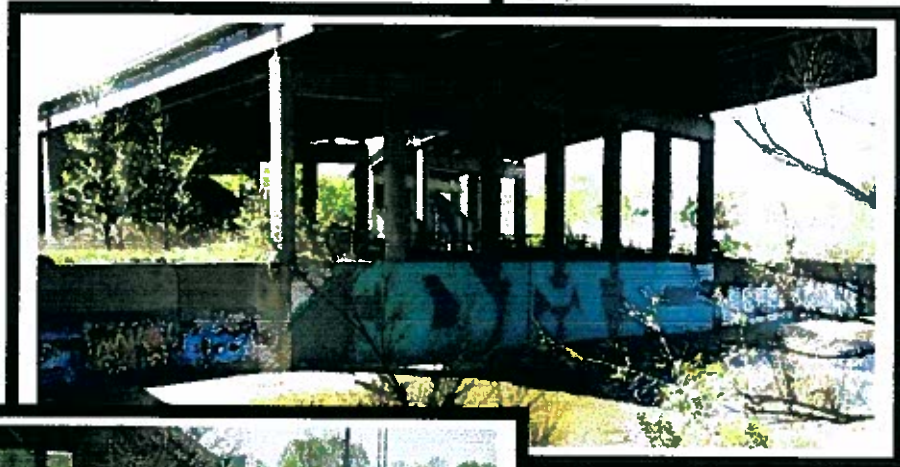
CPR BRIDGE B-10 MILE POST 88
