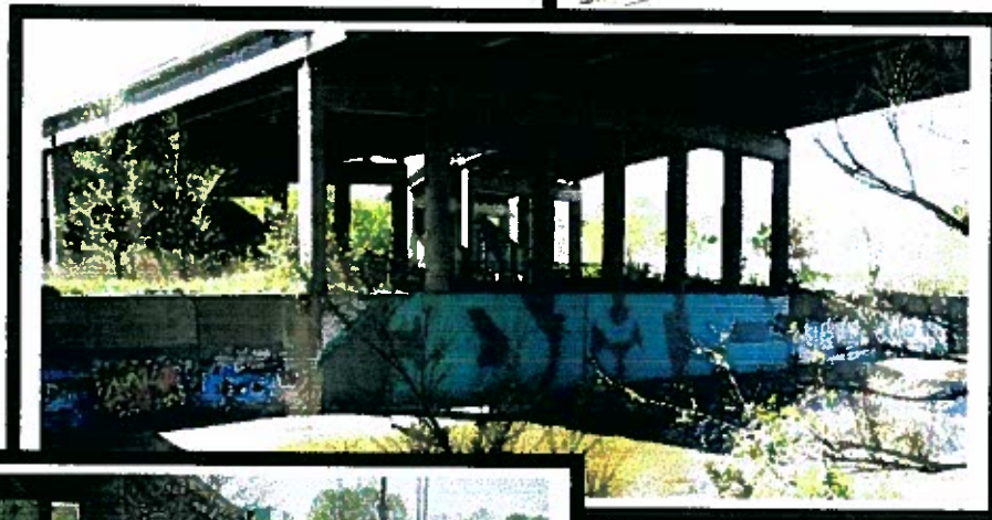
CPR BRIDGE B-10 MILE POST 88
