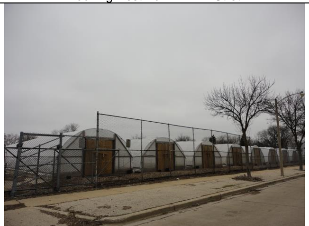
Looking westerly from N. 41 st Street
