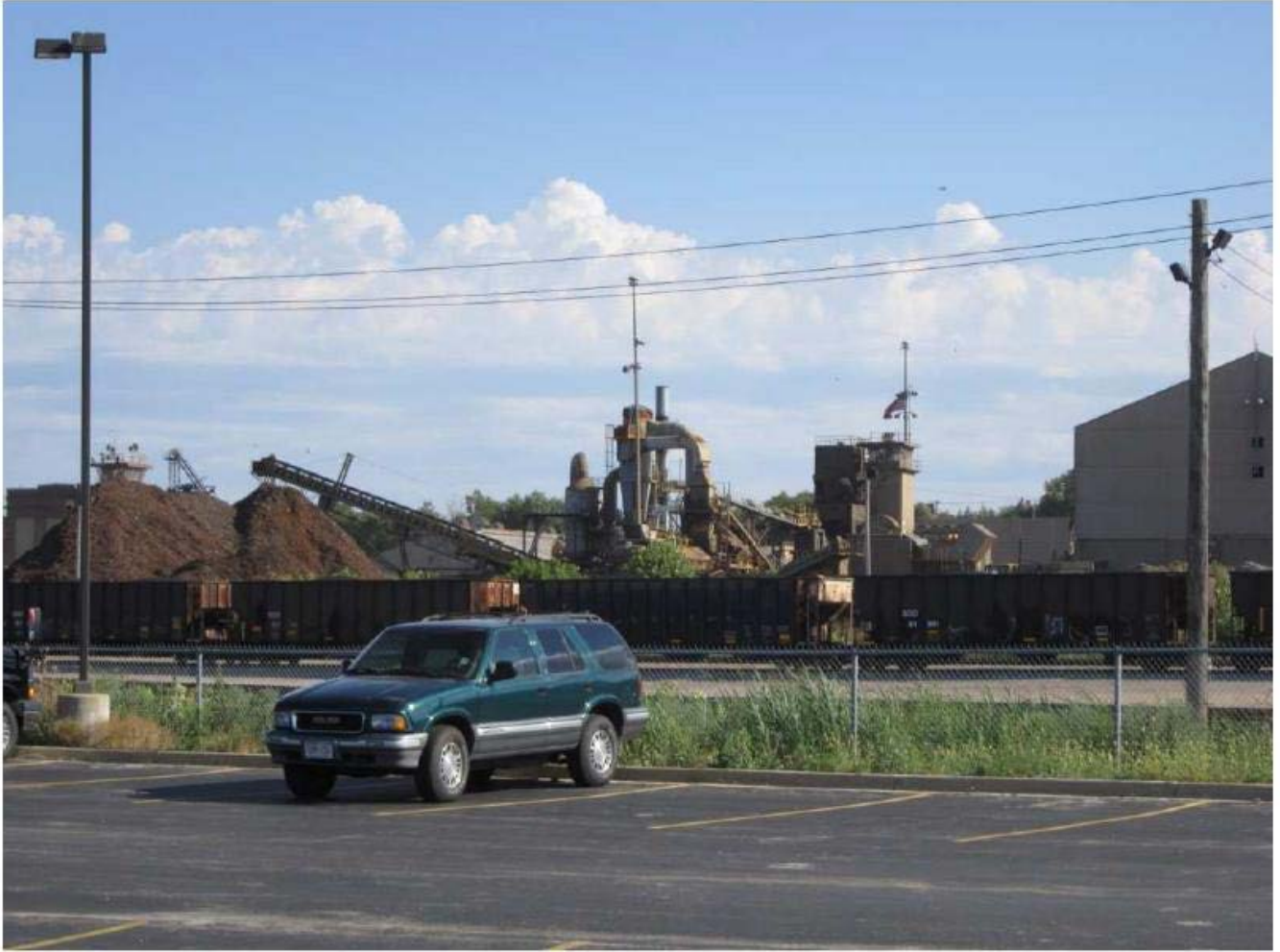
South View from Biogas Generation Site
