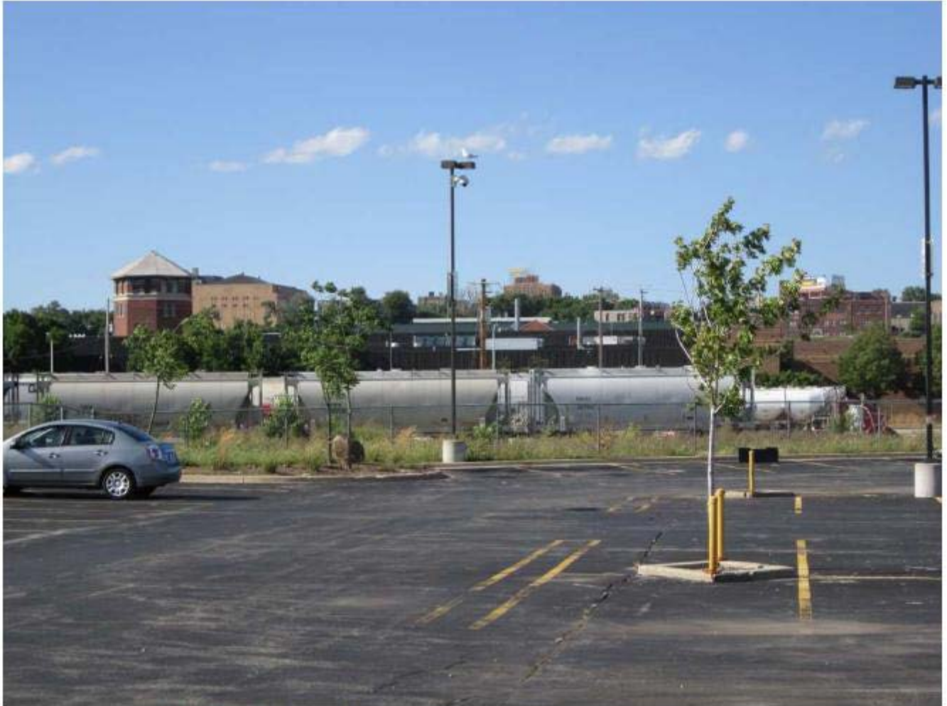
North View from Biogas Generation Site
