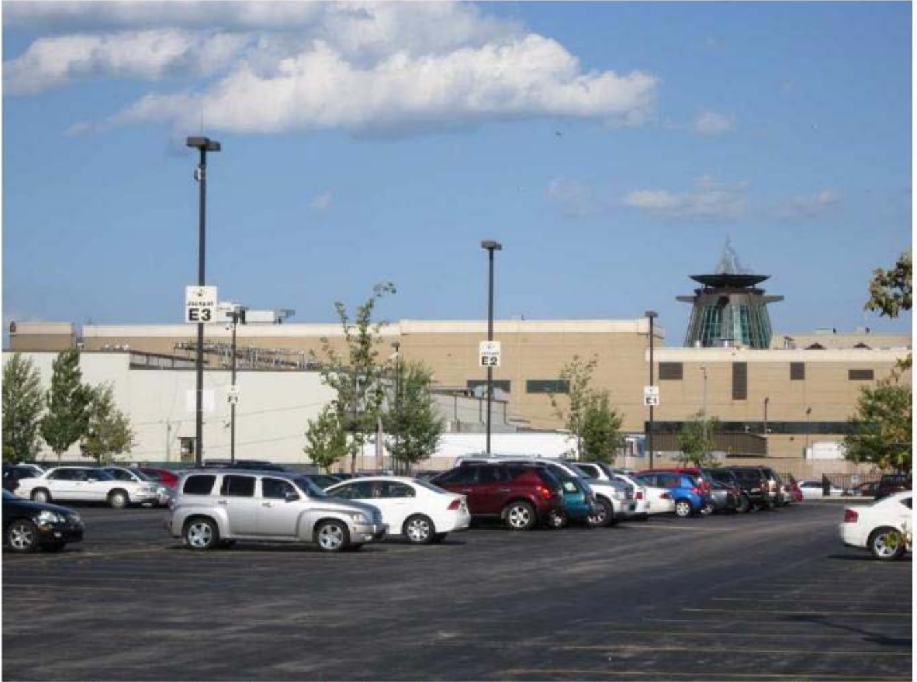
East – Northeast View from Biogas Generation Site
