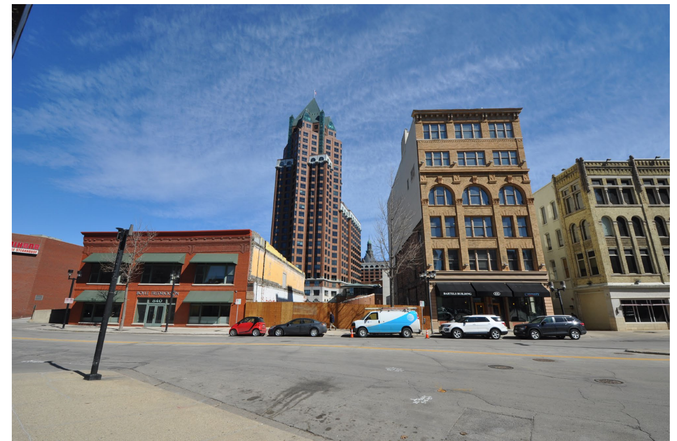
Front of Site - Plankinton Side
