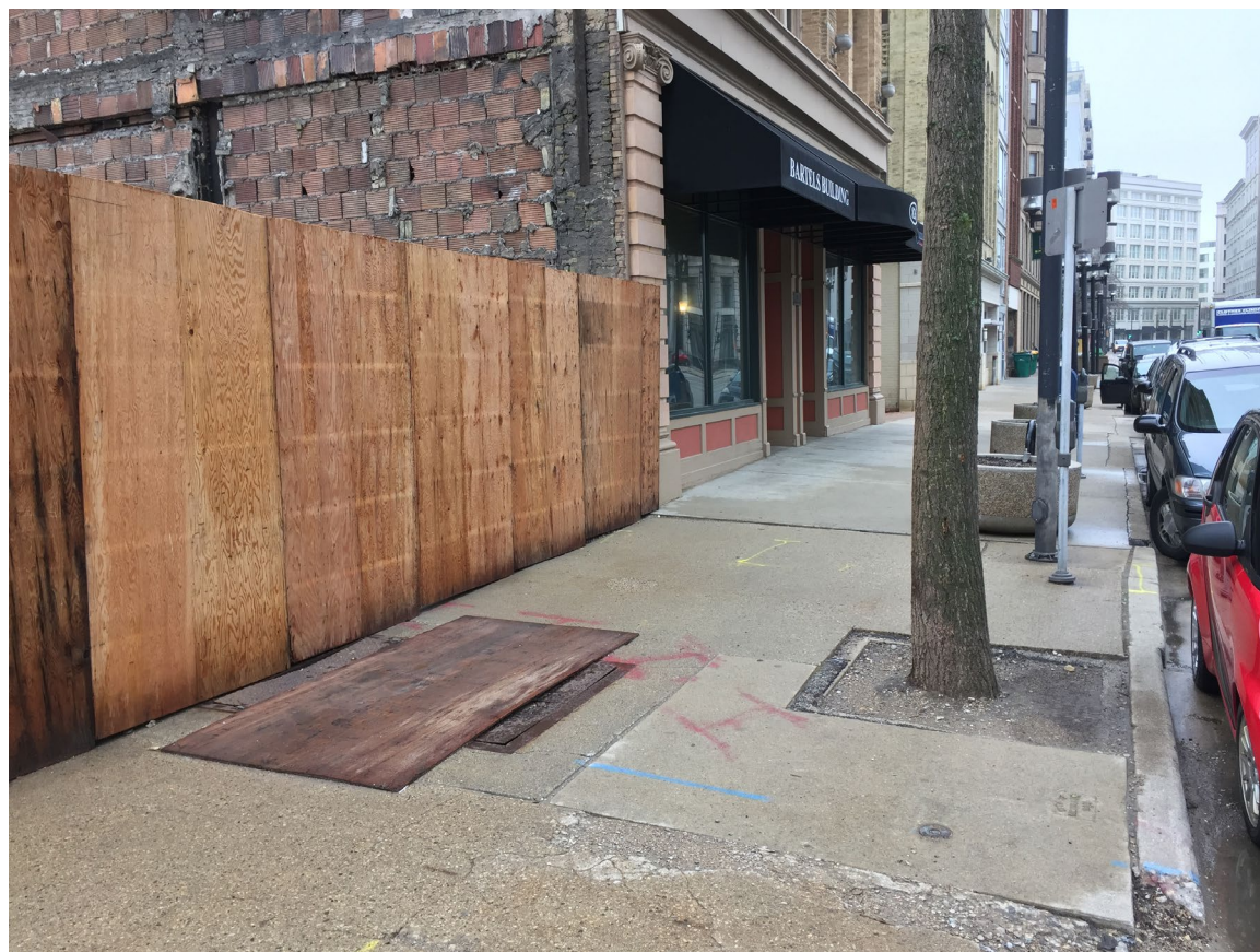
Sidewalk on Plankinton - Looking South
