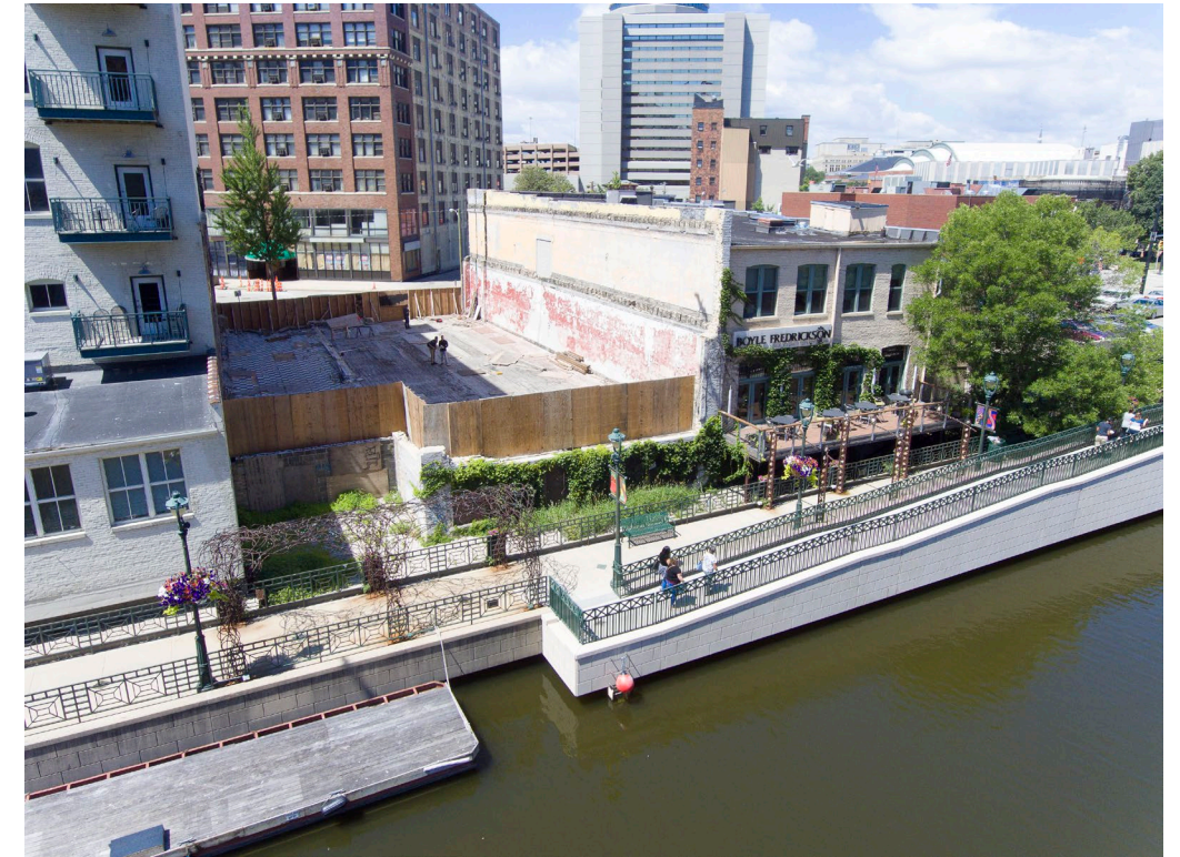
Rear of site - River Side
