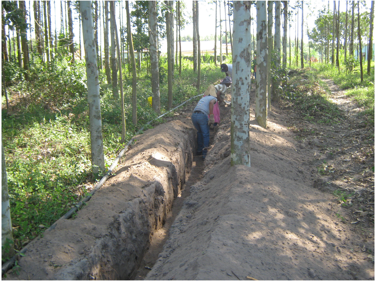
Women backfilling the trench by hands using a spade
