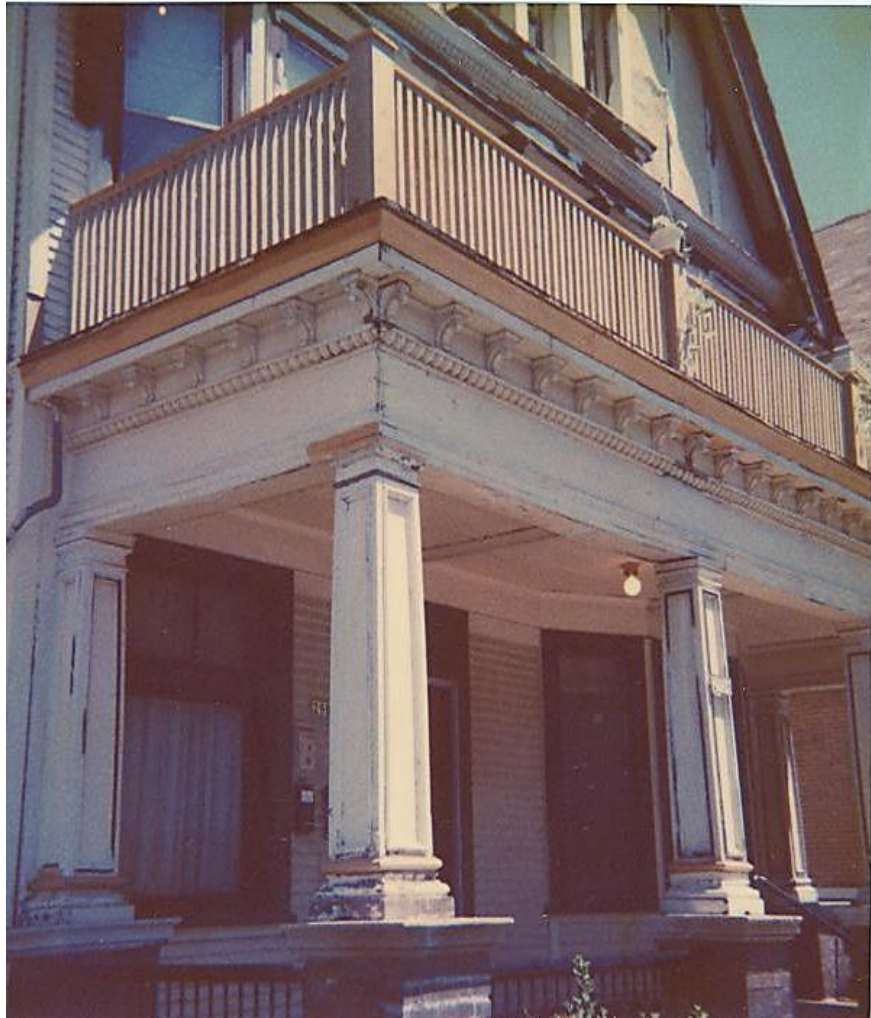
Deteriorated columns, date unknown (c. 2007).
