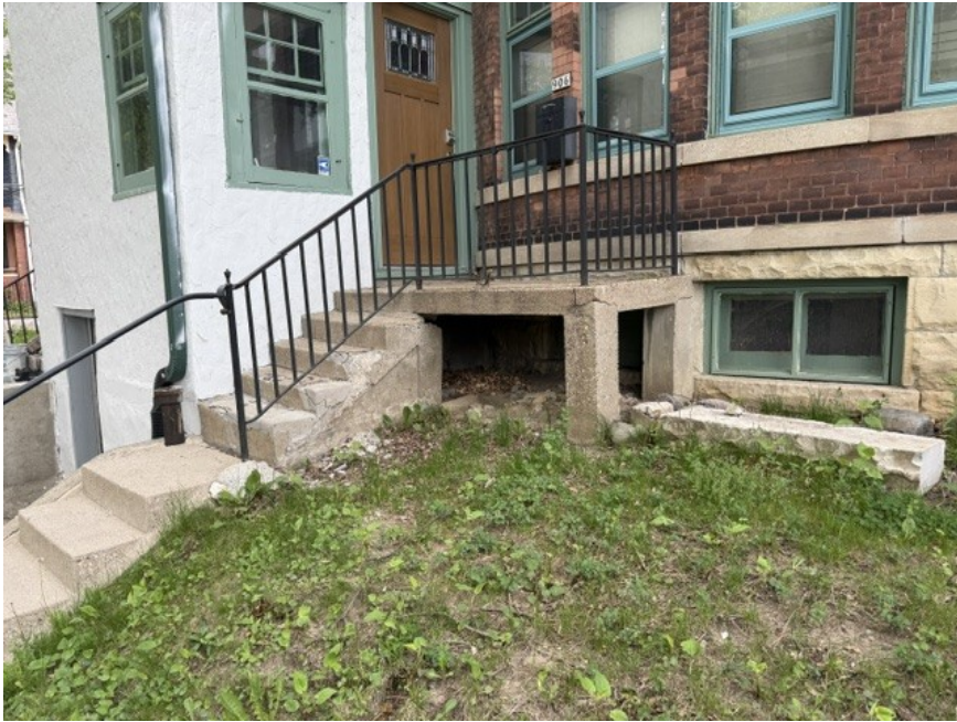
Existing porch and step condition
