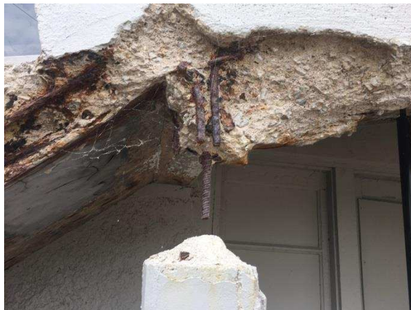
Photo 'C': Top of Column
