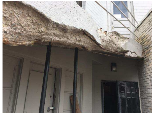
Photo 'D': Edge Beam of Landing
