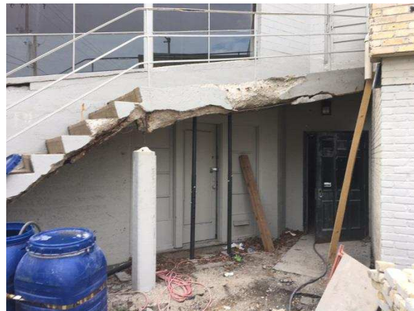
Photo 'B': West Elevation of Stairs
