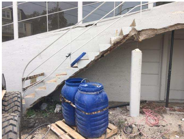
Photo 'A': West Elevation of Stairs
