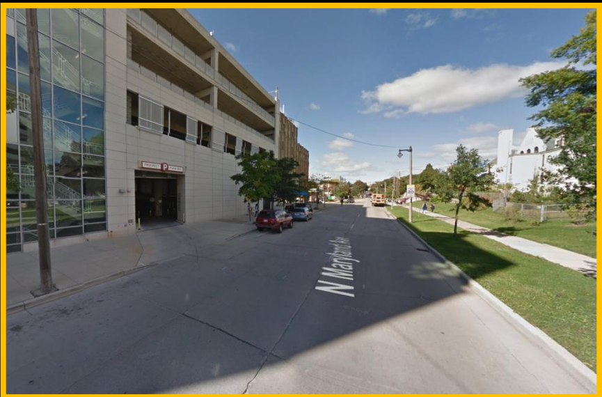
View from North Maryland Avenue, looking north
