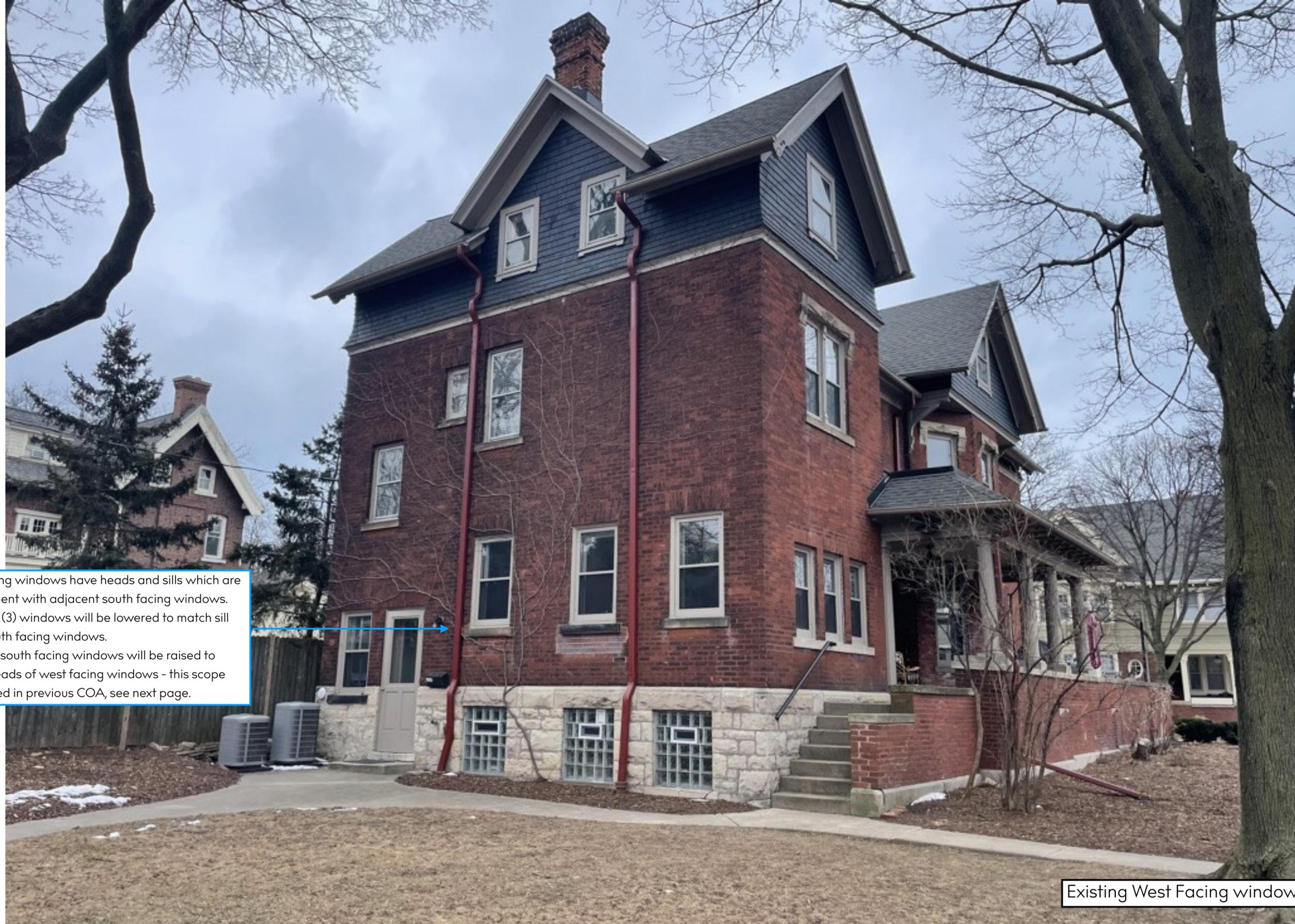
(3) West facing windows have heads and sills which are not in alignment with adjacent south facing windows. Sills of these (3) windows will be lowered to match sill height of south facing windows. Heads of (3) south facing windows will be raised to align with heads of west facing windows - this scope was approved in previous COA, see next page.
