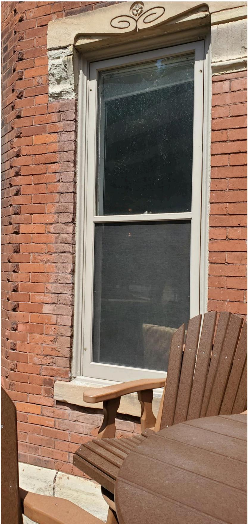
Photograph of existing wood storm windows. on this home. New storm windows for the west facing windows will match color and profile
