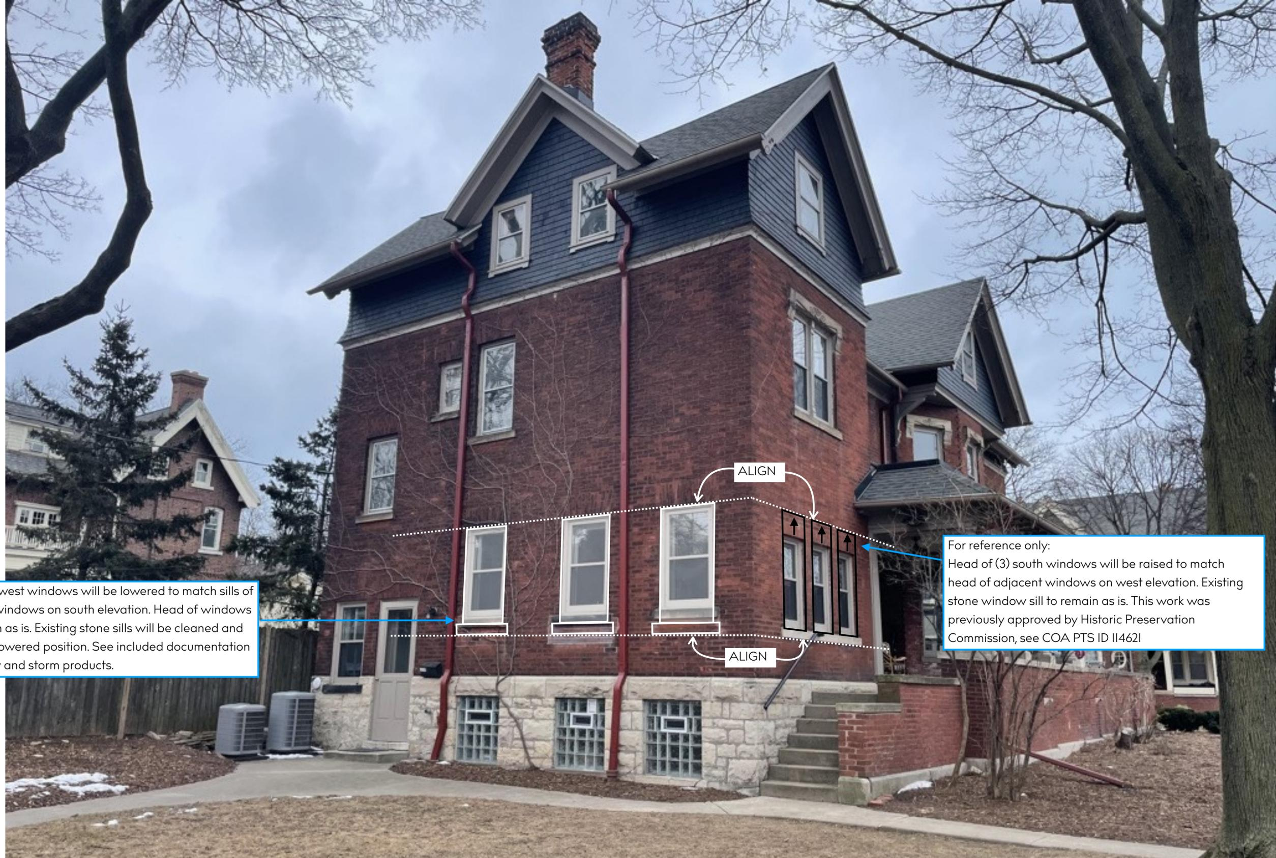
Sills of (3) west windows will be lowered to match sills of adjacent windows on south elevation. Head of windows will remain as is. Existing stone sills will be cleaned and reused in lowered position. See included documentation of window and storm products.
