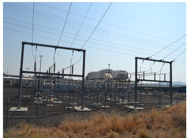
Google Data Center, The Dalles, Oregon, USA — High-voltage transmission lines feed directly into on-site substations, converting grid power to the stable, continuous electricity required to run thousands of servers. Photo by Visitor7 (Wikimedia Commons).
