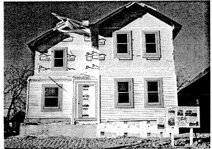
NEW CONSTRUCTION 1430 W. Chambers
