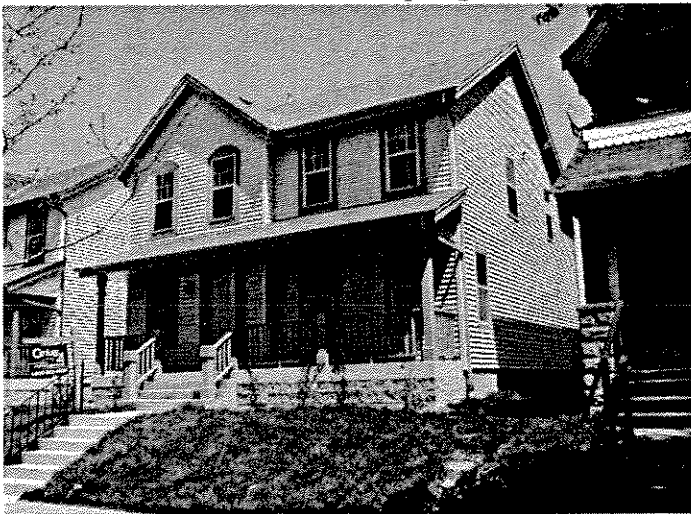
NEW CONSTRUCTION 15 th & Center
