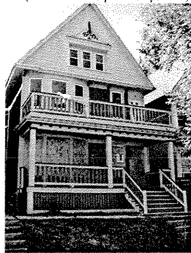
HOUSING REHABILITATION 34 th and North Avenue (West End Development Corporation)
