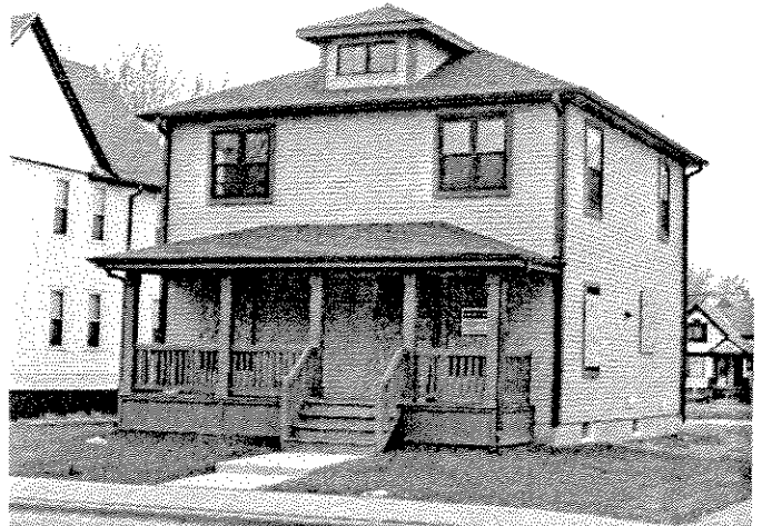
NEW CONSTRUCTION 2118 N. 27 th Street (Neighborhood Improvement Development Corporation)
