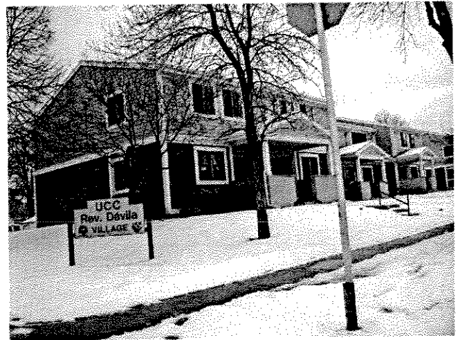
LA CASA DAVILLA REHABILITATION 8 th and Washington (United Community Center & Friends of Housing)
