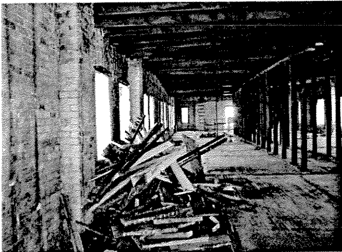
MATAYAS BUILDING RENOVATION 2443 N. Holton Street
