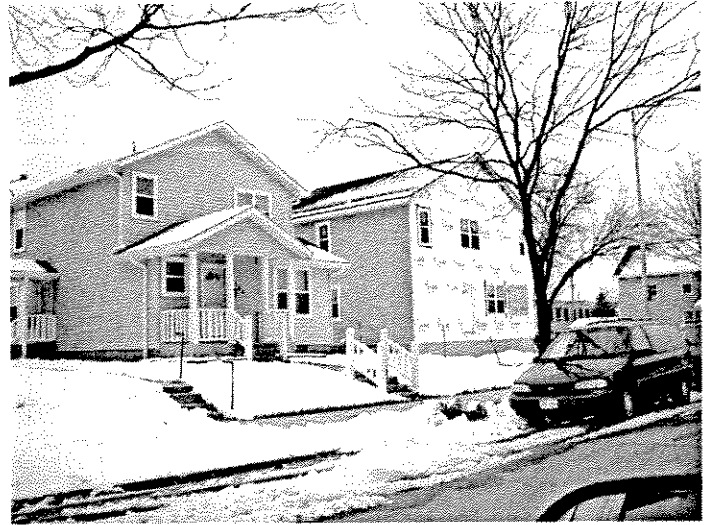
NEW CONSTRUCTION – FRESH START 28th and Vine (Howard Fuller Educational Foundation)
