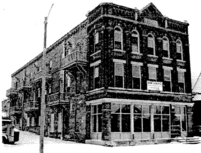
MATAYAS BUILDING RENOVATION 2443 N. Holton (Wisconsin Preservation Fund)
