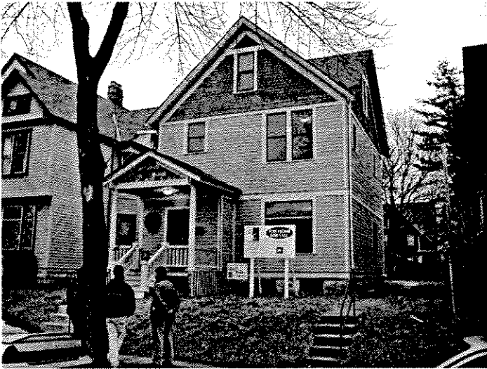
HOUSING REHABILITATION 34 th and North Avenue (West End Development Corporation)
