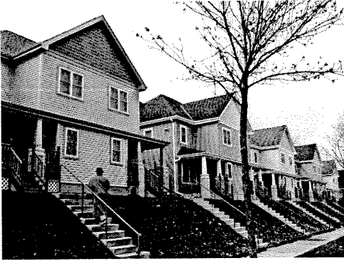
LEON SULLIVAN TOWNHOMES 3200 Block of North 2 nd Street (scattered sites) (Inner City Redevelopment Corporation)
