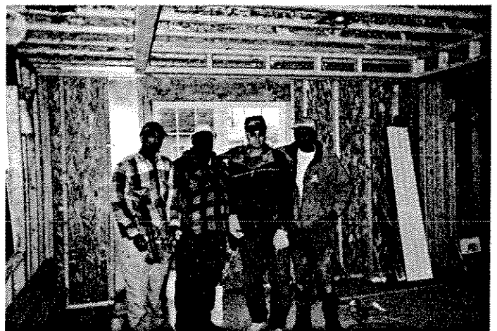
NEW CONSTRUCTION – FRESH START 28th and Vine (Howard Fuller Educational Foundation)
