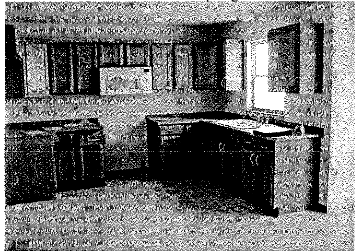
NEW CONSTRUCTION 15 th & Center
