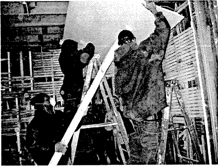
HOUSING "GUT" REHABILITATION 2432-34 N. 36 th Street (Milwaukee Community Service Corps)
