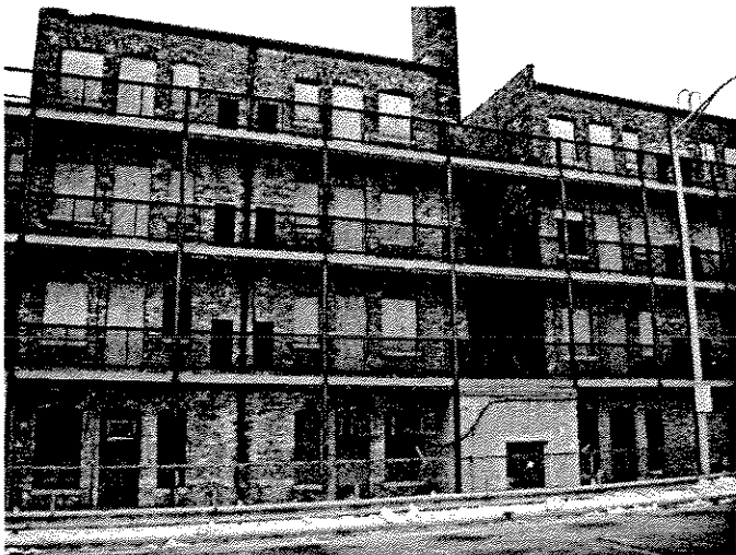
WEST POINTE CONDOMINIUMS (IN PROGRESS) 27 th and Wells Street (West End Development Corporation)
