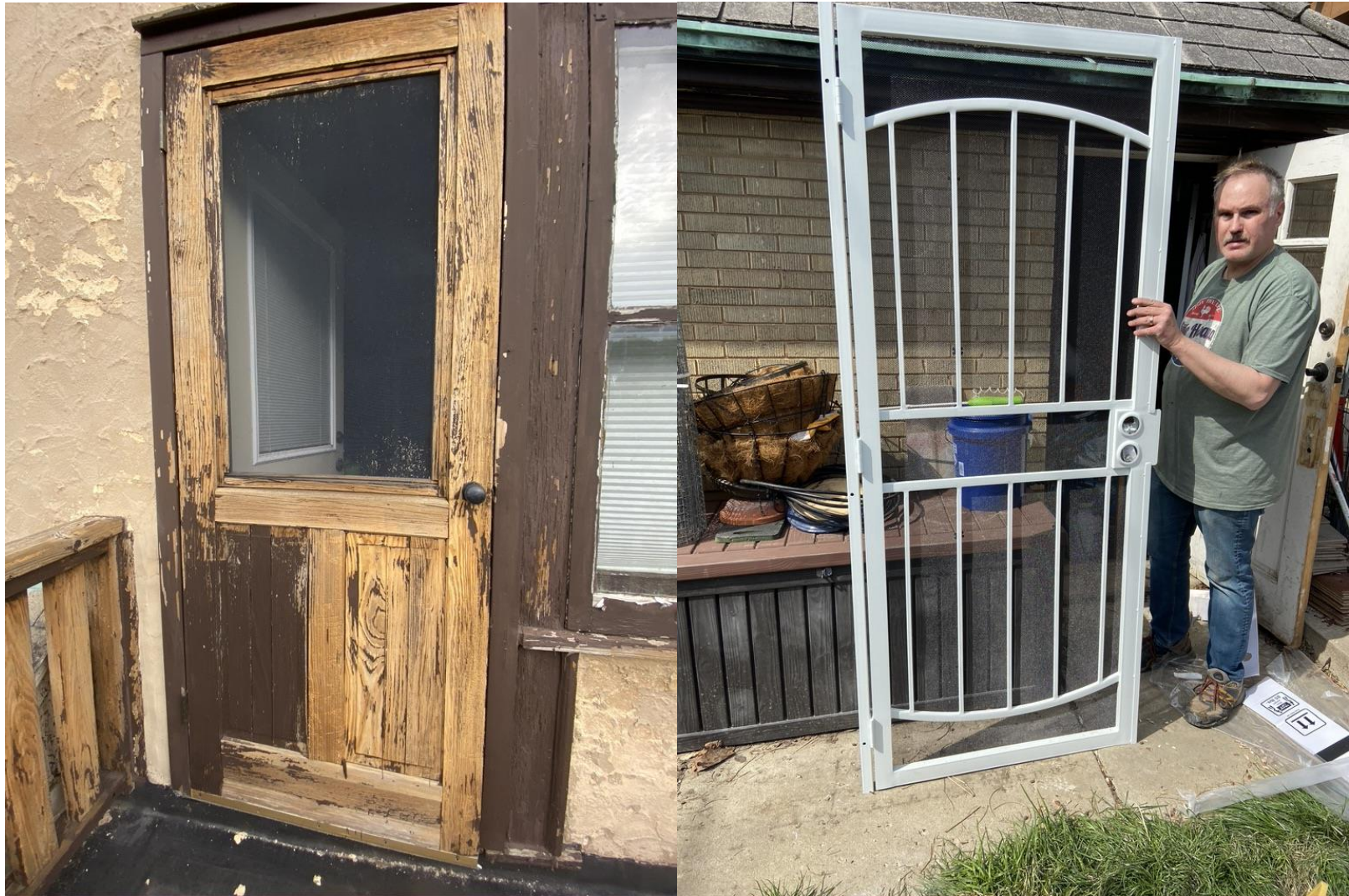
Existing and replacement doors. New security door must be painted to match surrounding building materials.
