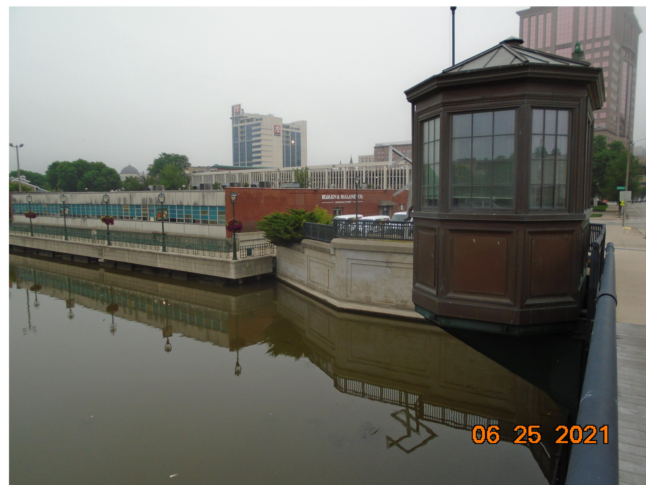
EXISTING RIVERWALK I IMAGE
