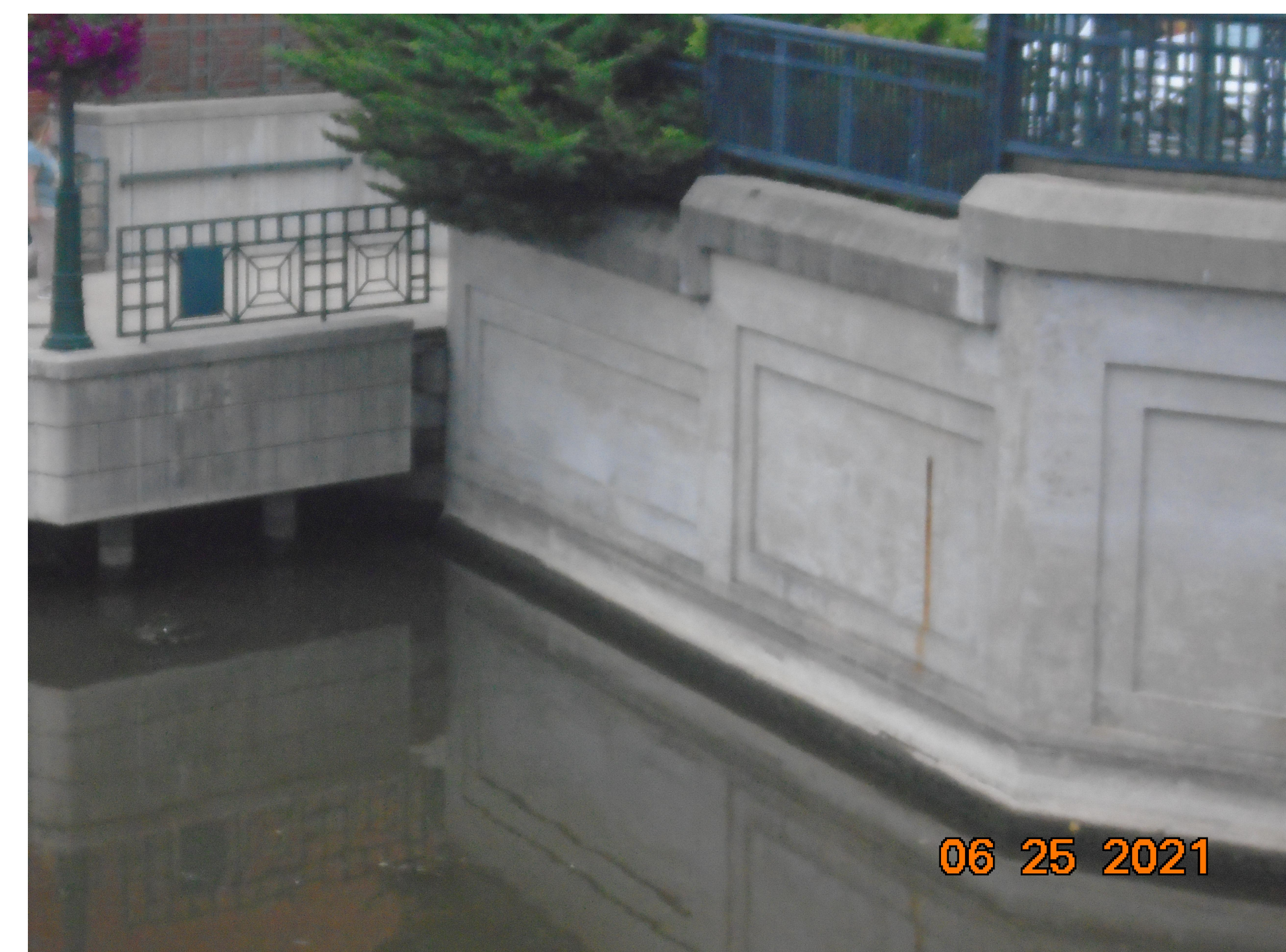
EXISTING RIVERWALK I IMAGE
