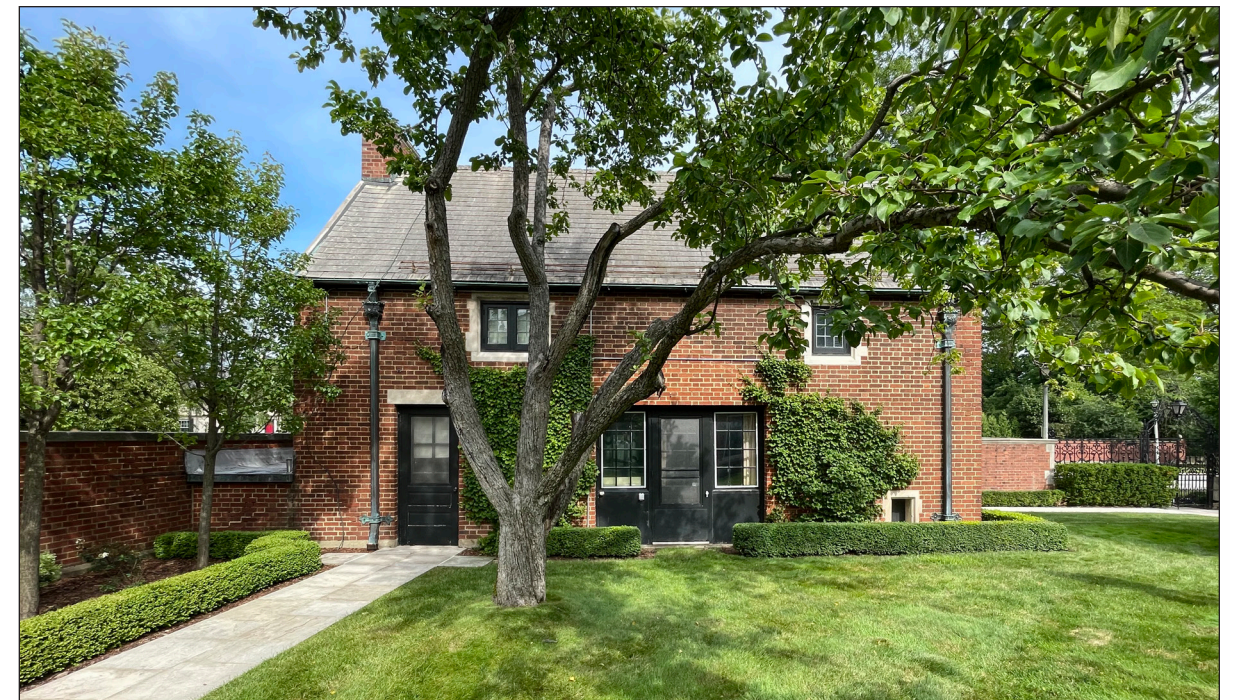
Caretaker's Cottage - West Elevation
