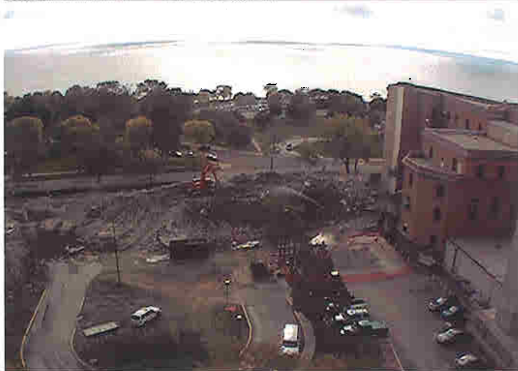
SITE OF FORMER 1958 HILL BUILDING – PROPOSED WTMC BLDG.
