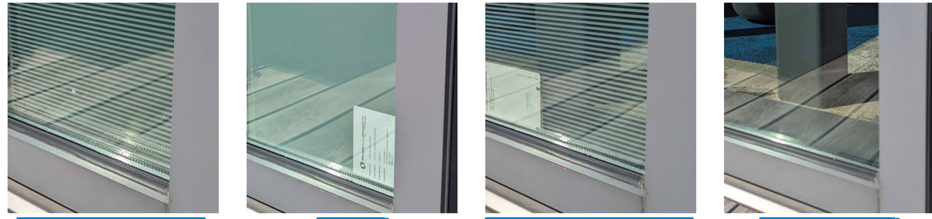
SPANDREL GLASS WITH LINEAR FRIT PATTERN (50% COVERAGE) FROSTED GLASS OBSCURED LOW-E INSULATING VISION GLASS WITH LINEAR FRIT PATTERN (50% COVERAGE) LOW-E INSULATING VISION GLASS
