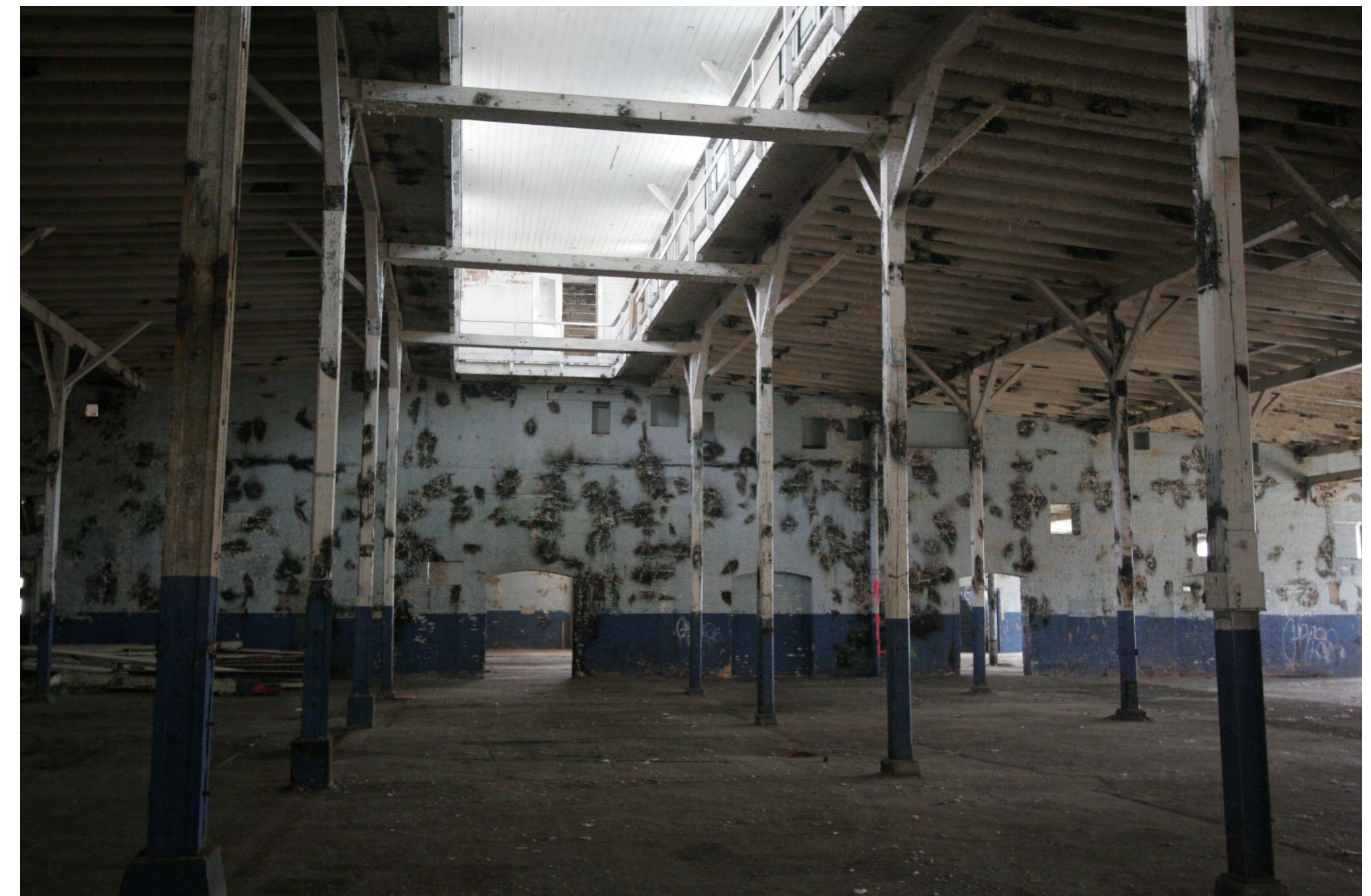
LEVEL 2 - CENTER OF BUILDING - NORTH LIGHT MONITOR
