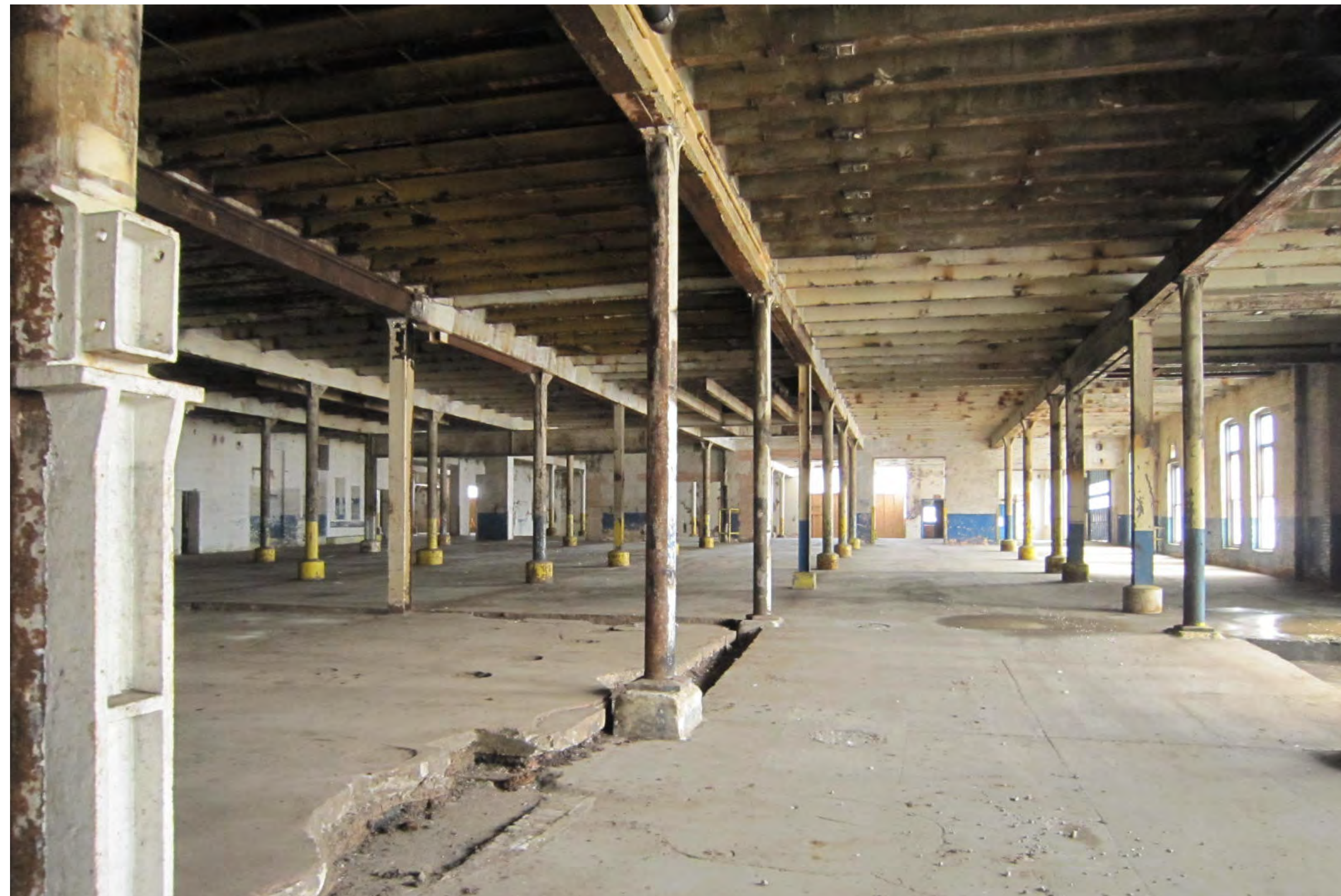
LEVEL 1 - ALONG SOUTH WALL
