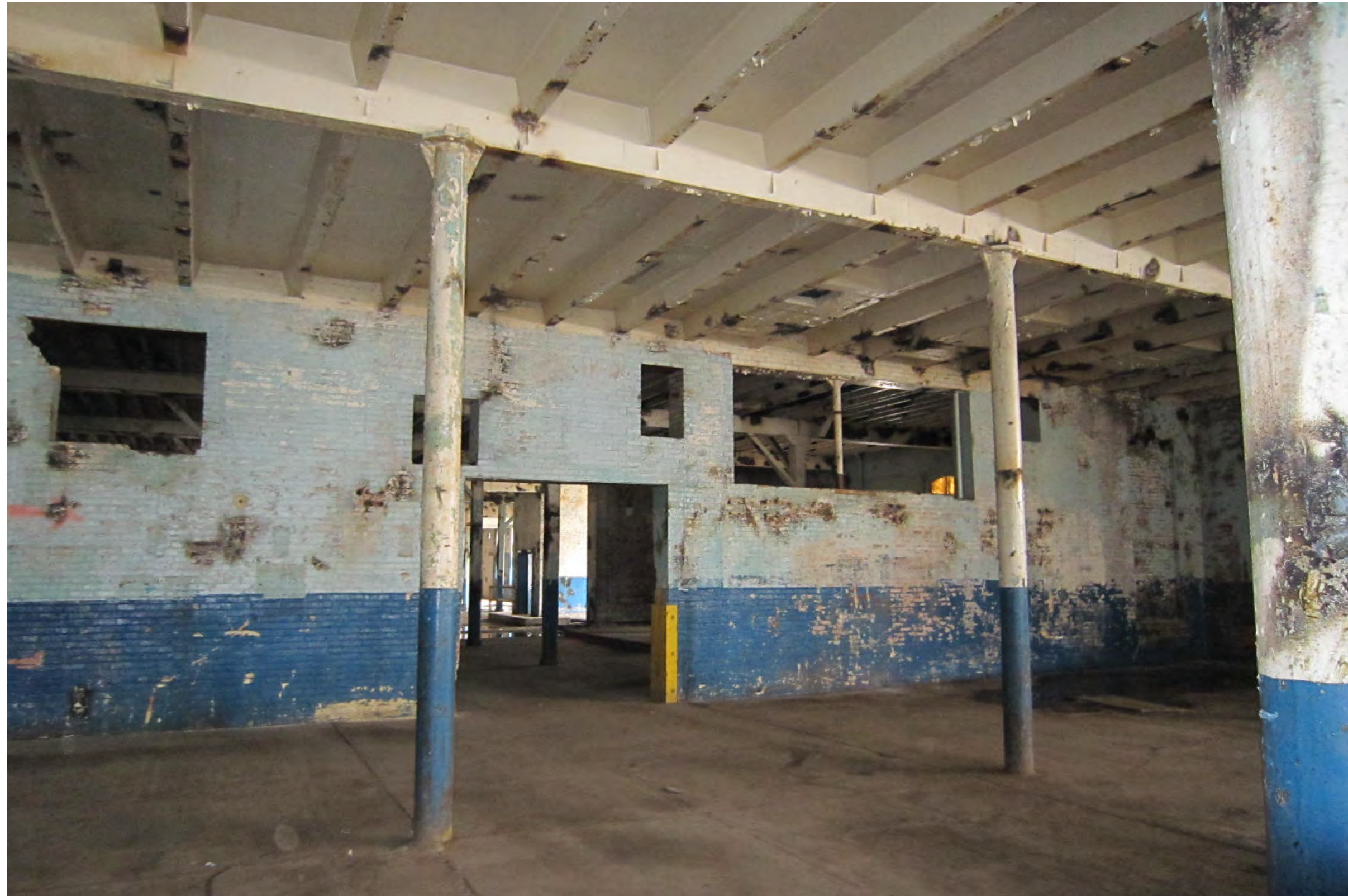
LEVEL 2, EAST SIDE - LOADING DOCK AREA
