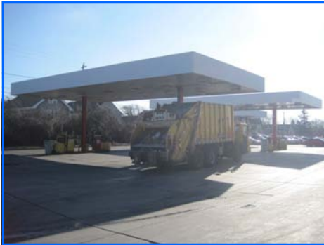
Fuel Island structures
