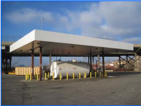
Fuel island and storage tank
