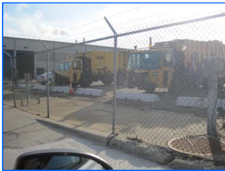
Chain link fence with barbed wire
