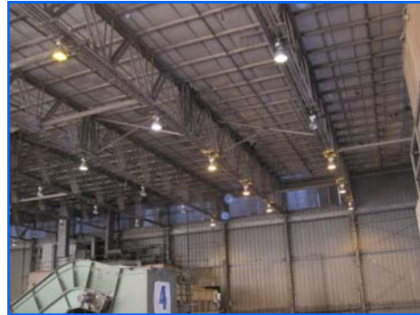
Typical pendulum light fixtures attached to roof truss
