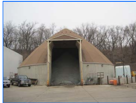
Salt dome with asphalt shingle roof
