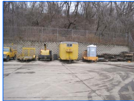
Chain link fence with barbed wire - note retaining wall
