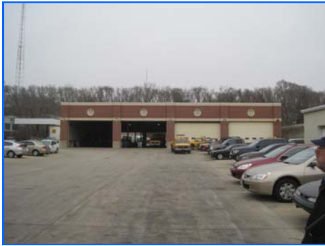
Typical condition of concrete
