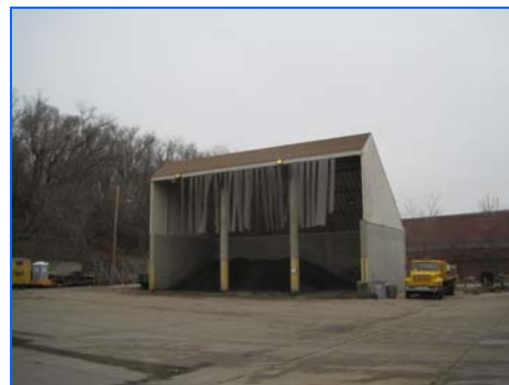
Soil shed with asphalt shingle roof
