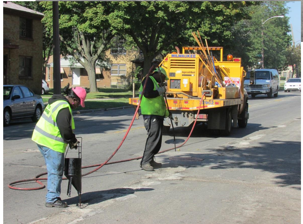
Pothole filling and patching
