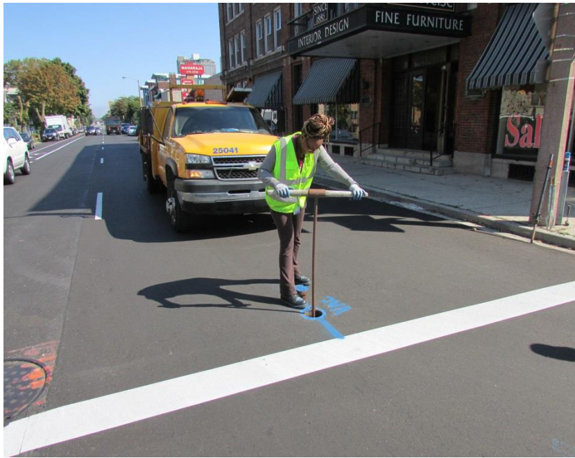
Exercising a water main valve
