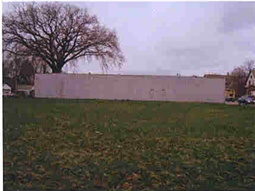
View of the project site from the South.
