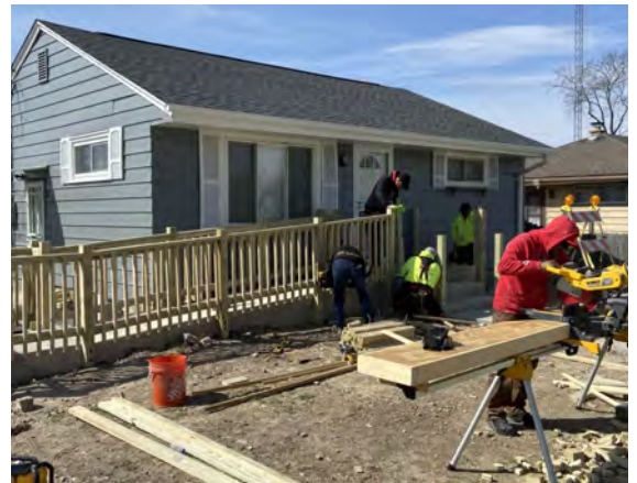
Rehab in progress with accessible entryway.
