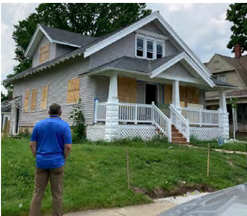
Team member reviews renovation.
