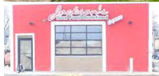
"Before and After" on West Fond du Lac Avenue.
